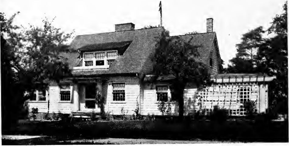
RESIDENCE FOR MRS. S. E. FENTON, EAST CLEVELAND DERCUM & BEER, ARCHITECTS, CLEVELAND
