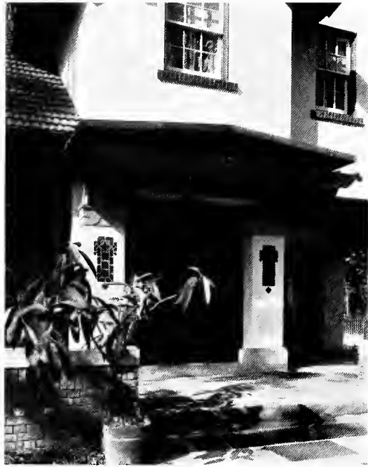
RESIDENCE OF MR. TROXEL, ELYRIA, O. GEO. H. STEFFENS, ARCHITECT, J. F. STEFFENS, DESIGNER, CLEVELAND.
