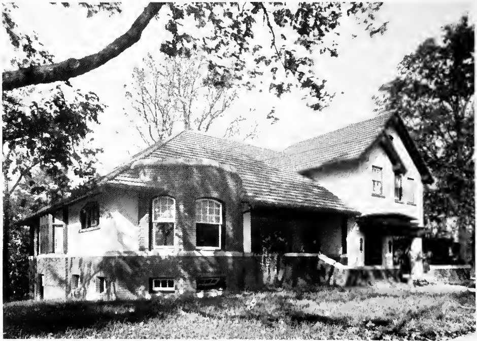
RESIDENCE OF MR. TROXEL, ELYRIA, O. GEO. H. STEFFENS, ARCHITECT, J. F. STEFFENS, DESIGNER, CLEVELAND.
