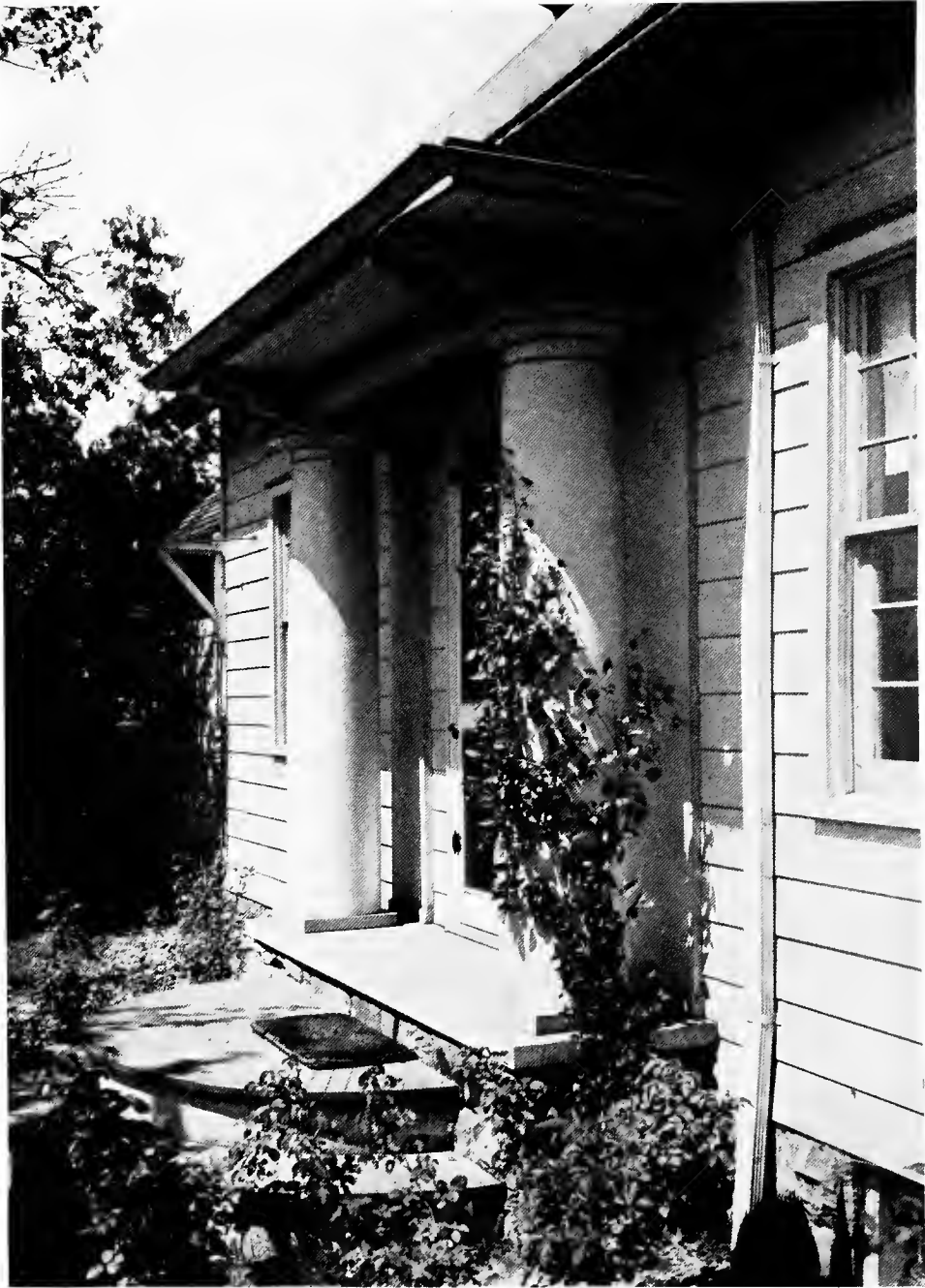
ENTRANCE DETAIL HOUSE IN EAST CLEVELAND DERCUM & BEER, ARCHITECTS, CLEVELAND
