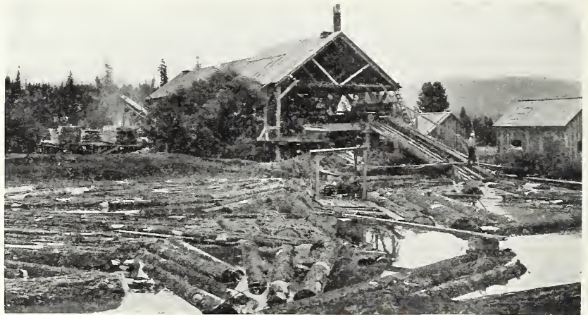
FIGURE 28.—Circular sawmill in western Washington having a capacity of approximately 30,000 board feet per 8-hour shift. The chief products of small mills are railroad ties, planking, timbers, common boards, and dimension. Usually such mills are located in the woods near their log supply
