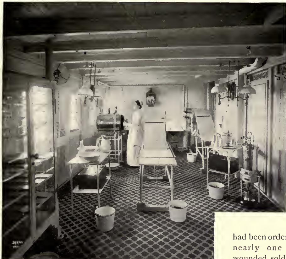
THE OPERATING-ROOM OF THE RELIEF
