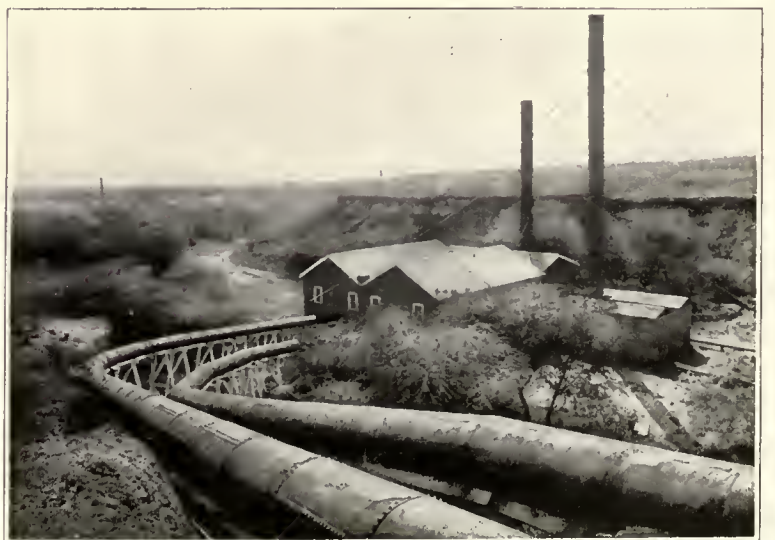
SUGAR-PLANTATION PUMPING-STATION IN HAWAII
