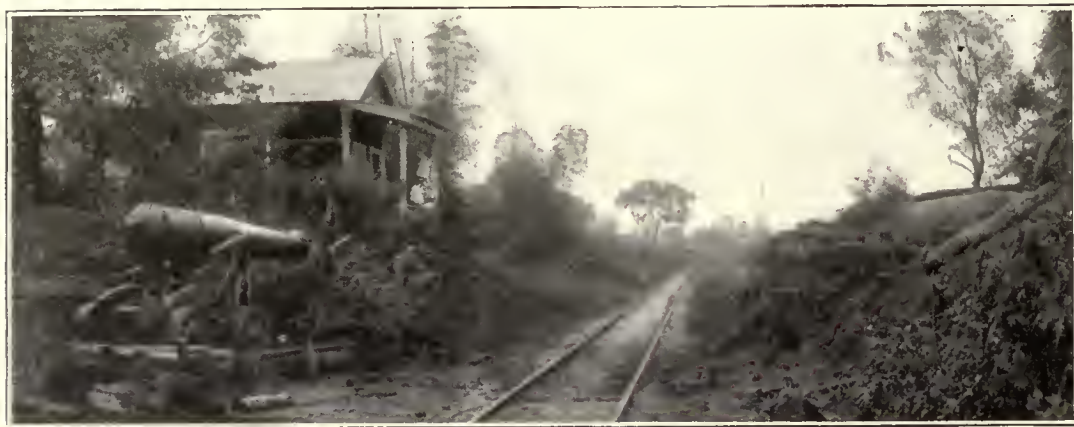
GUN MOUNTED BY INSURGENTS TO CONTROL THE RAILROAD NEAR CALOOCAN
