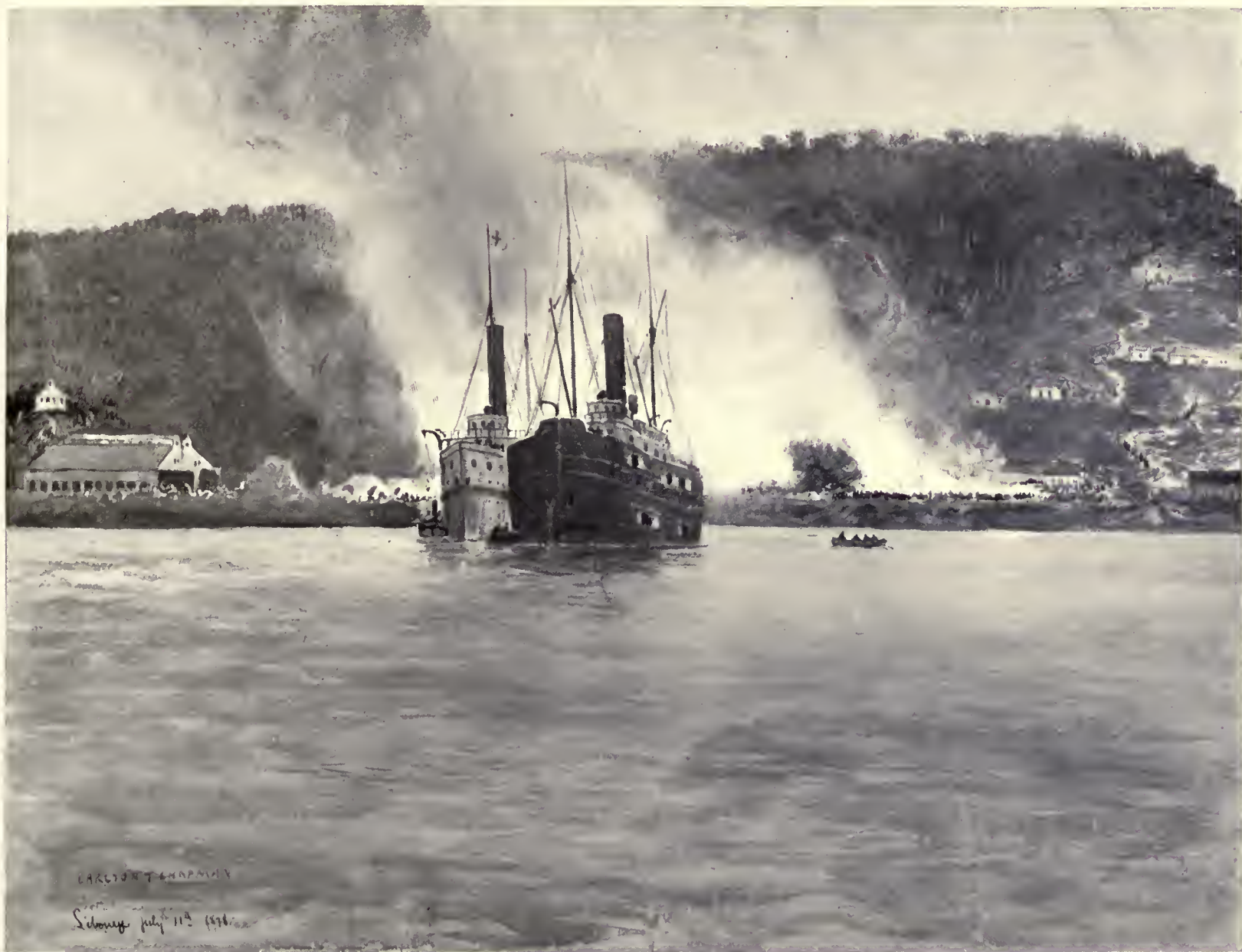
Block-house Railroad Round-house
