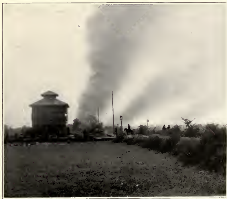
BLOCK-HOUSE No. II, LOOKING TOWARDS SAN PEDRO MACATI
