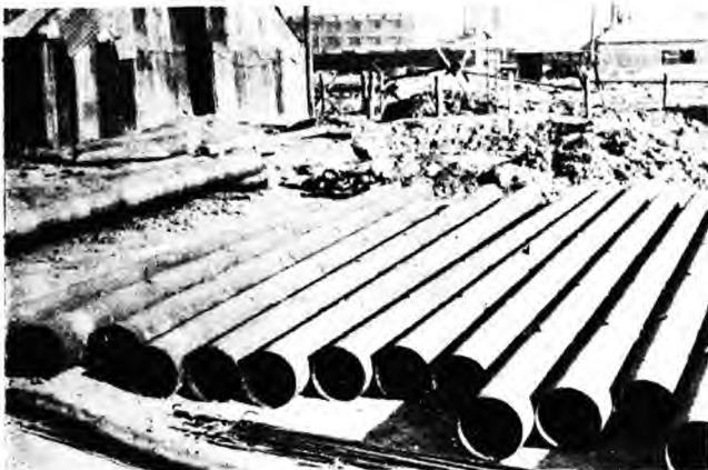
WELL CASING FORMED FROM TANK PLATE READY FOR PLACING
