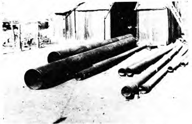
PRELIMINARY 20" DIAMETER ROUGH CASING READY FOR PLACING.
