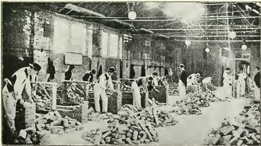
Brick-laying Department—Students at Work, New York Trade School.
