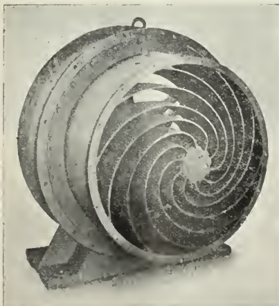
Fig. 2.—Schlotter-blower with free shaft-end. View of the guide blades.
