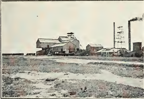
The South Rand Colliery at Grootvlei.
