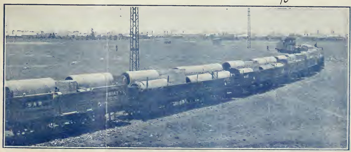
TEN TRUCK LOADS OF PIPES LEAVING FACTORY FOR WYNBERG, C.P.
