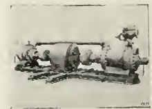
SULZER MINE PUMP
