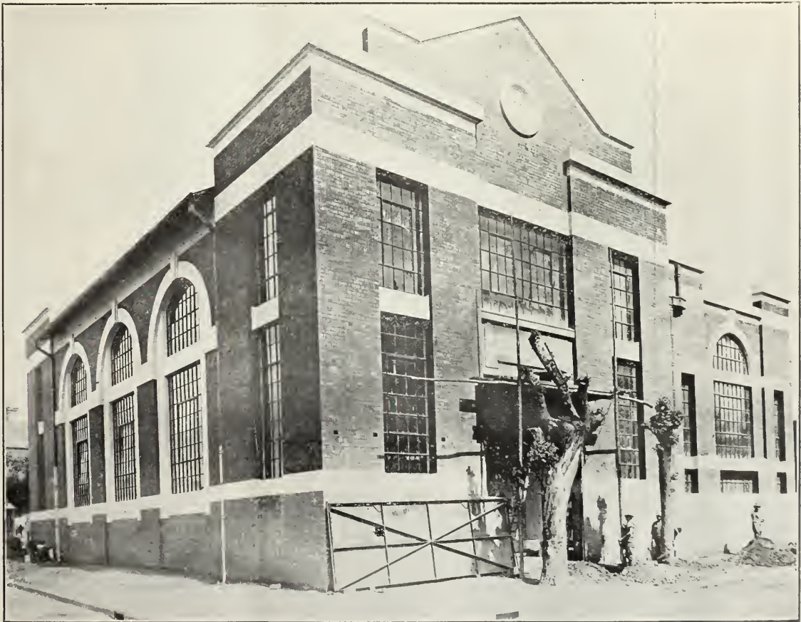
New Municipal Power Plant Sub-Station.
