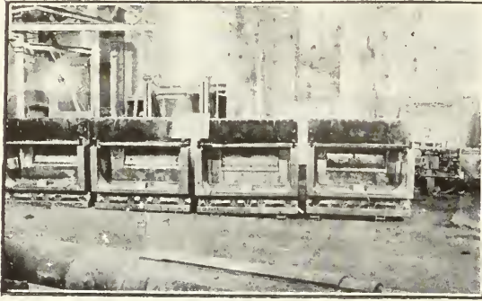
Mcrtar Boxes for Robinson Deep, turned out by Tarry's.
