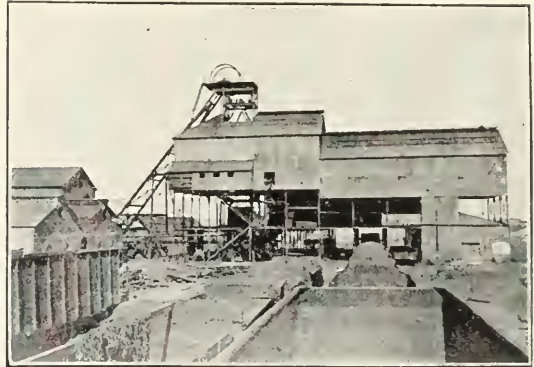
South Rand Colliery—Headgear and Screening Plant.
