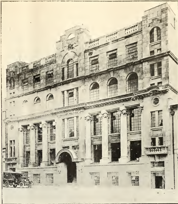
A Large and Palatial Warehouse just completed in Market Street.
