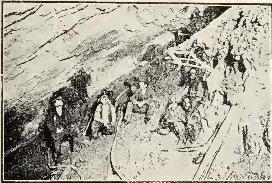
Underground on a Rand Mine.
