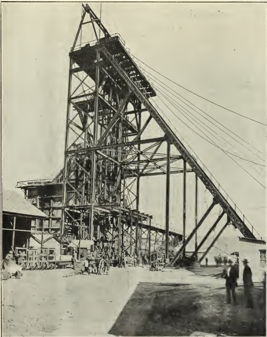
A New Photograph of the Headgear at the Turf Shaft, the Deepest Shaft on the Rand. Idle on account of the Strike, which has now lasted for more than a month.
