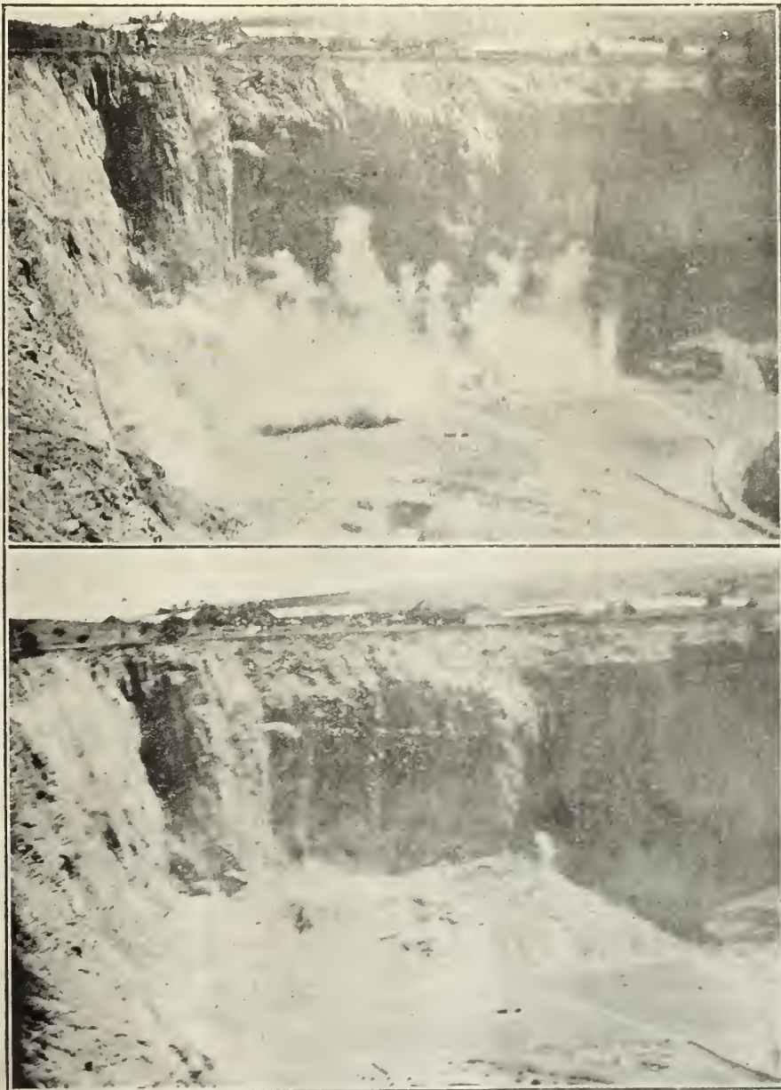
(1) A Blast at the Premier Mine. (2) What it Brought Down.
