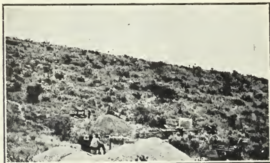
Opening up a Diamond Mine near Postmasburg.
