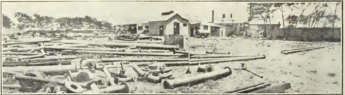
General View of the Works.
