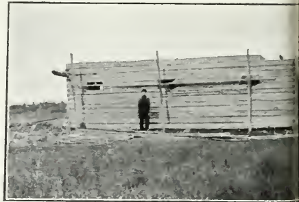
AN OLD COMMUNITY STABLE BEING REBUILT ON AN INDEPENDENT'S HOMESTEAD.
