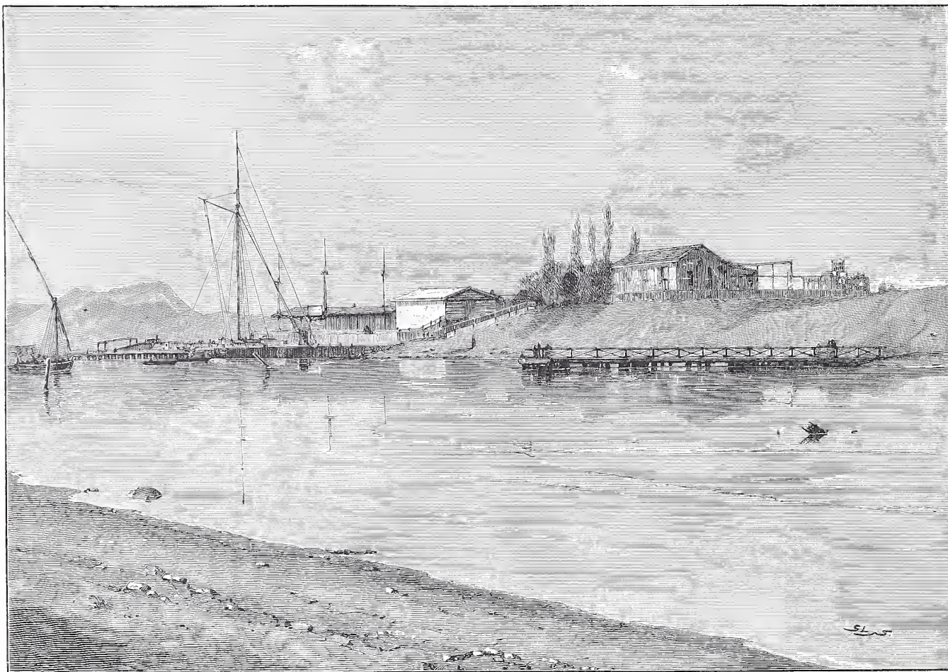
The Station at Kantarah, on the Suez Canal.
