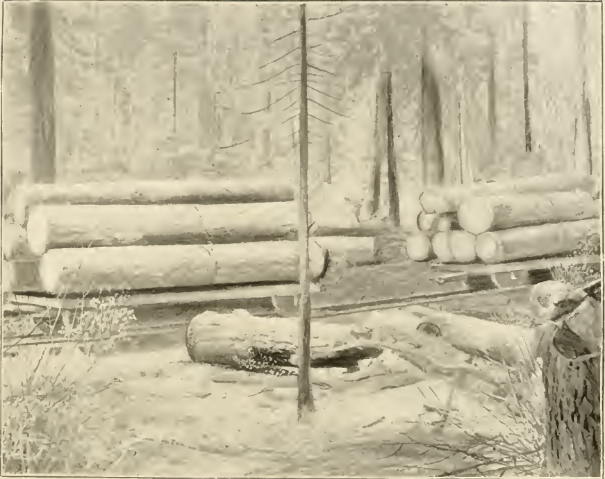
.1. LOGGING TRACKS AND LOAD, NEAR SNOW, T. 40 S., R. 5 E.
