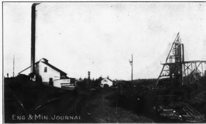
POWER PLANT AND HEADFRAME OF THE CUYUNA-MILLE LACS
