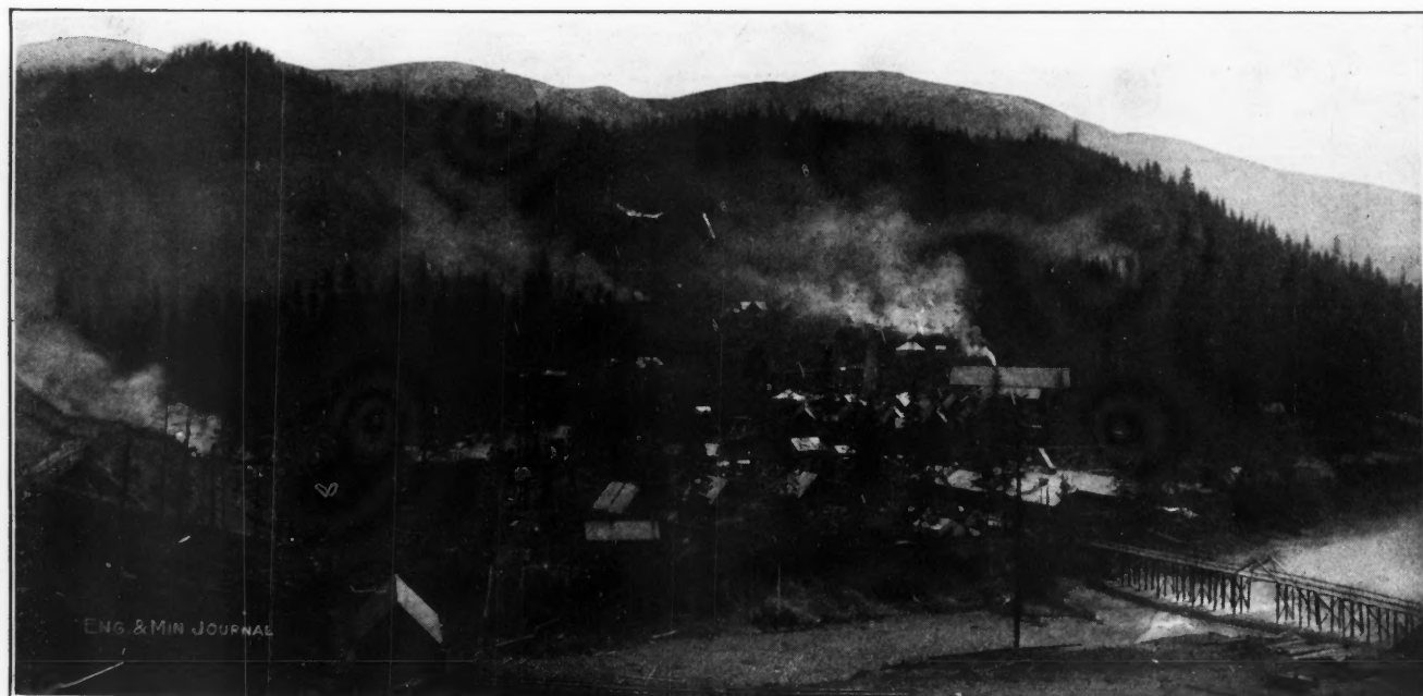
GENERAL VIEW OF TOWN OF ANYOX, B. C., FROM ORE-BIN SITE View as it appeared June 27. Granby company has built hotel, 100 cottages and other buildings, with all modern conveniences for housing about 600 smelter employees.
