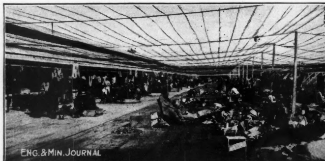
INSIDE OF THE KIMBERLEY COMPOUND
