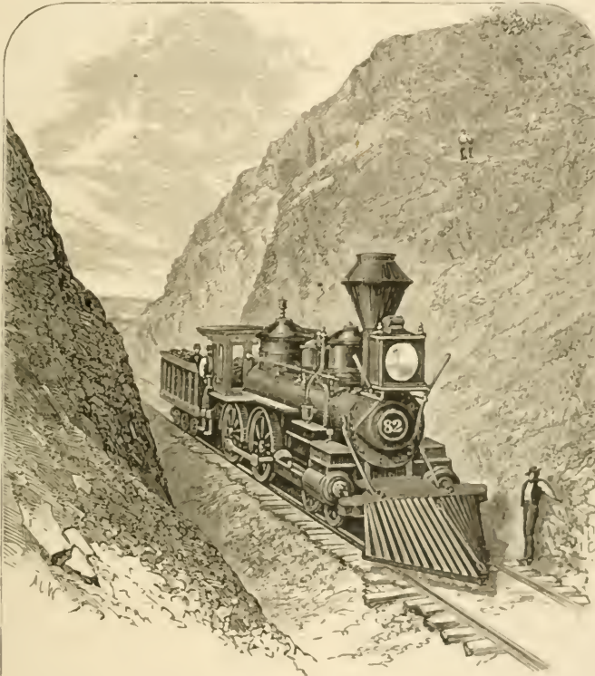
ROCK CUT, NEAR ASPEN.
