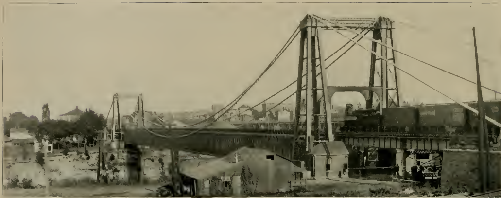
GRAND TRUNK SUSPENSION BRIDGE REPLACED BY STEEL ARCH BRIDGE IN 1897.
