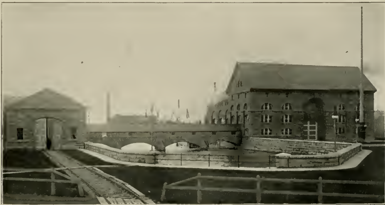
POWER HOUSE AND TRANSFORMER HOUSE, NIAGARA FALLS POWER COMPANY
