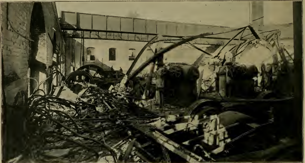
INTERIOR OF ENGINE ROOM—UNION TRACTION COMPANY, PHILADELPHIA.
