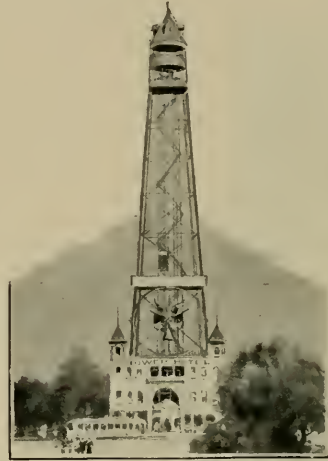
TOWER OWNED BY GORGE ROAD.
