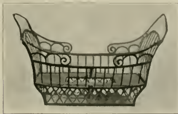
BASKET FOR CABLEWAY.
