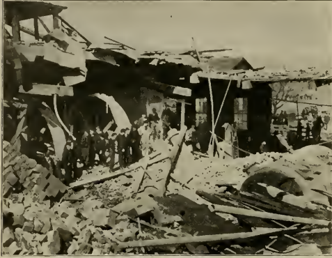
INTERIOR OF STATION.
