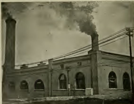
FIG. 8.—EXTERIOR OF STATION.
