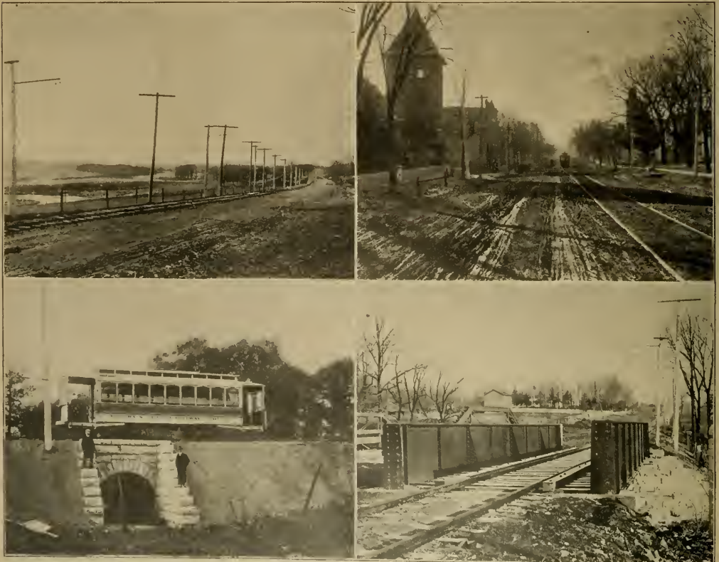
SCENE ALONG FOX RIVER. CULVERT AND CAR AT SULLIVAN'S CREEK, TWO MILES FROM AURORA.
