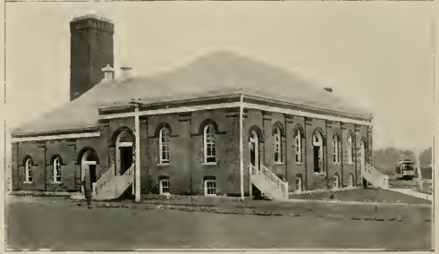
POWER HOUSE—MARION CITY RAILWAY.
