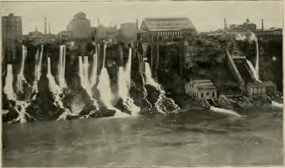
NIAGARA FALLS HYDRAULIC POWER & MANUFACTURING COMPANY.
