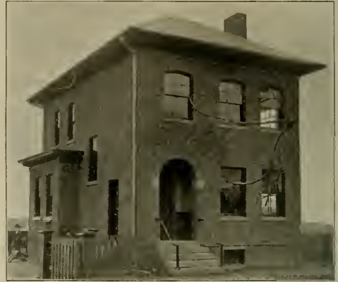
OFFICES OF THE FUEL ECONOMIZER COMPANY.
