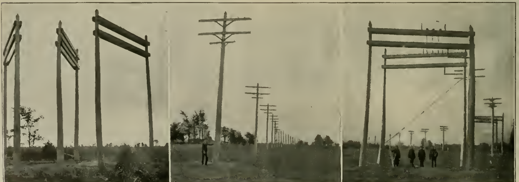
SAMPLES OF LINE CONSTRUCTION—NIAGARA FALLS-BUFFALO TRANSMISSION.
