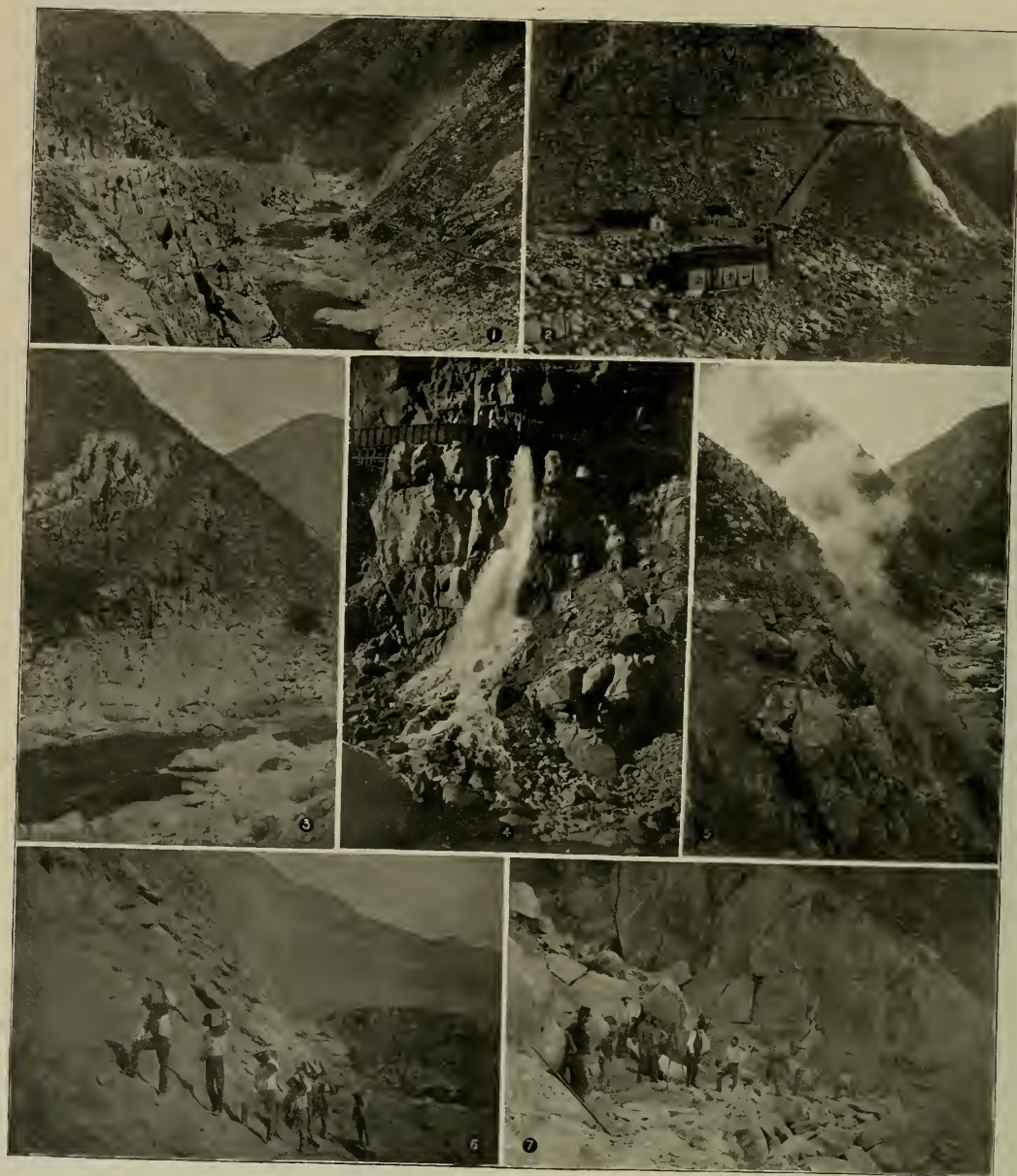
1—Looking up the river—the grade completed. 2—Panoramic view of power station. 3—Cañon before any work was done. 4—The safety gate. 5—Making the flume grade—just after a blast. 6—Carrying dynamite. 7—Making flume grade—in heavy stone.
