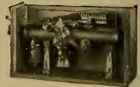
STANDARD AIR BRAKE AUTOMATIC REGULATOR.
