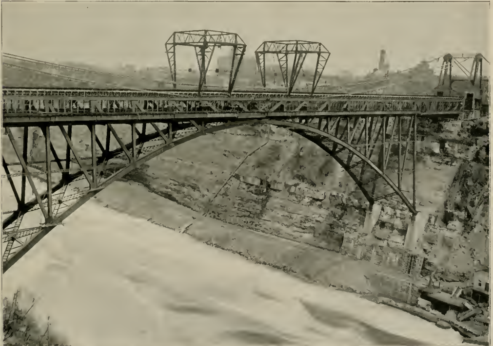
GRAND TRUNK DOUBLE DECKED STEEL-ARCH BRIDGE DURING CONSTRUCTION, 1897.
