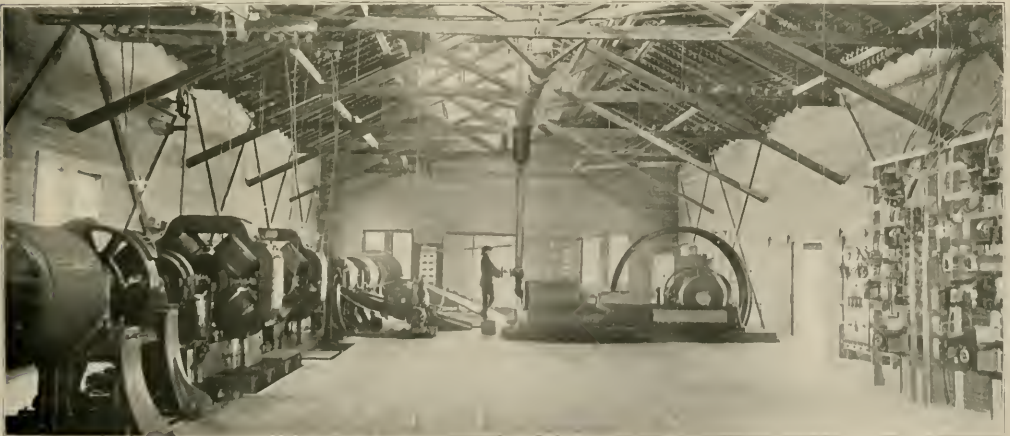
FIG. 2. INTERIOR OF POWER HOUSE, TAMPA, FLA.
