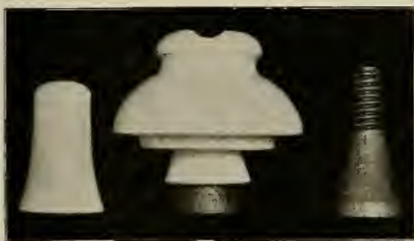
FIG. 2.—TWO PART INSULATOR.
