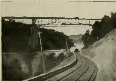
UNDER THE CANTILEVER BRIDGE.
