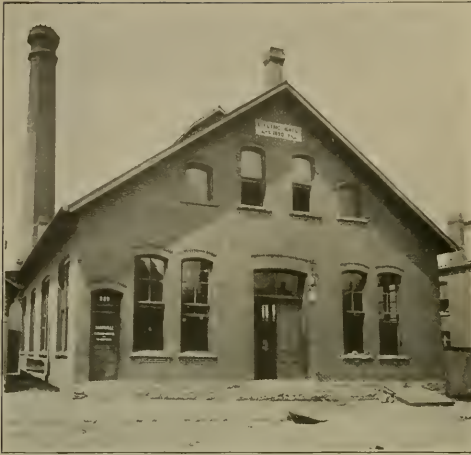
POWER STATION, ZANESVILLE, O.
