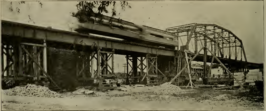
RAISING METROPOLITAN ELEVATED AT ROCKWELL STREET.
