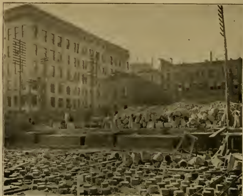
VIEW OF FOUNDATIONS.
