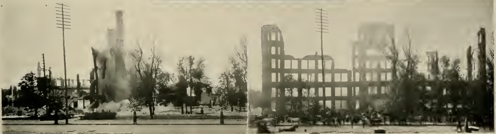
WRECKING WALLS WITH DYNAMITE.
