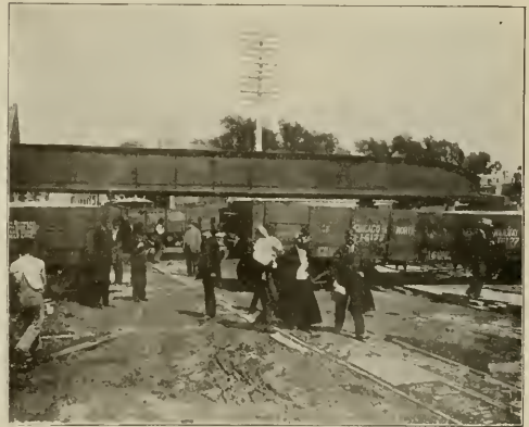
WEST CHICAGO TRACKS AT ROCKWELL STREET.
