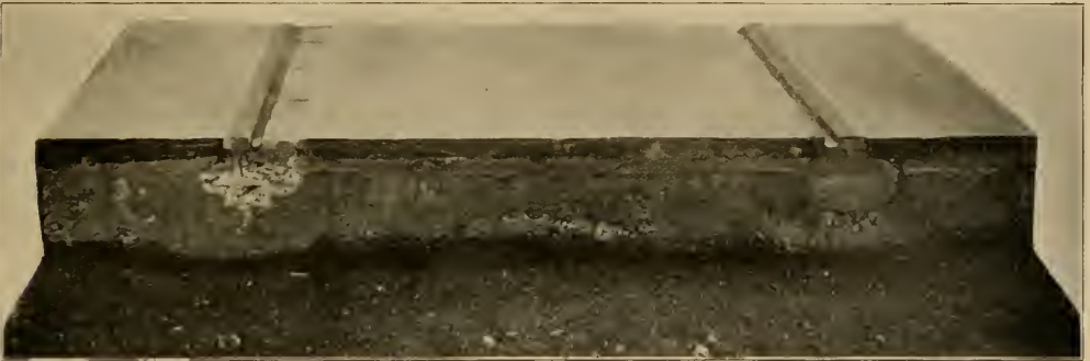
FIG. 2—SECTION OF TRENCH WORK—TWIN CITY RAPID TRANSIT COMPANY.
