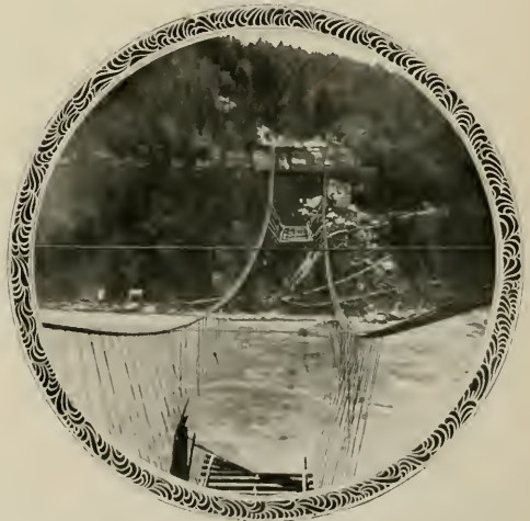
OLD BRIDGE AT LEWISTON.
