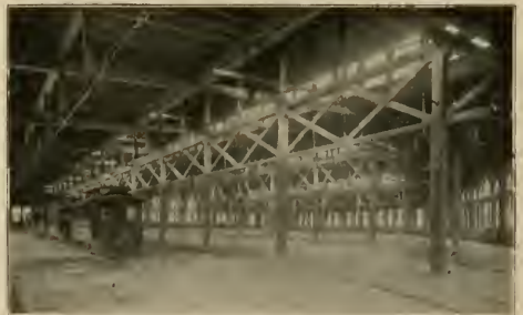
FIGURE 2—INTERIOR OF CAR HOUSE.
