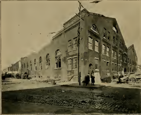
POWER HOUSE AFTER THE FIRE.
