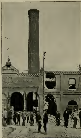
FIG. 1.—DAMAGED PORTION OF POWER HOUSE.
