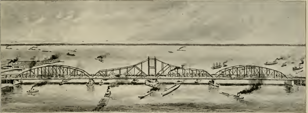
STEEL DRAWBRIDGE CONNECTING DULUTH, MINN., AND SUPERIOR, WIS.
