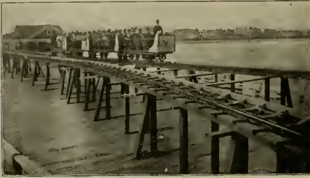
OCEAN PIER RAILWAY.
