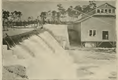
FIG. 1.—DAM AND POWER HOUSE.
