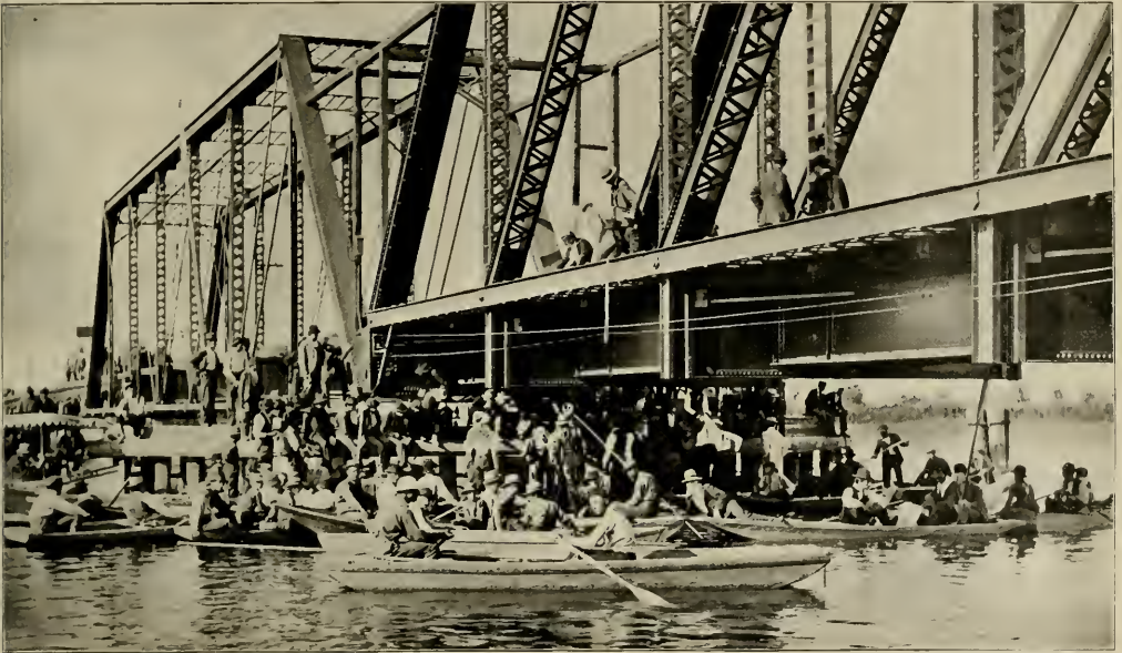
SCENE OF THE BRIDGE ACCIDENT, NEAR SAGINAW, MICH.—DIVERS AT WORK.
