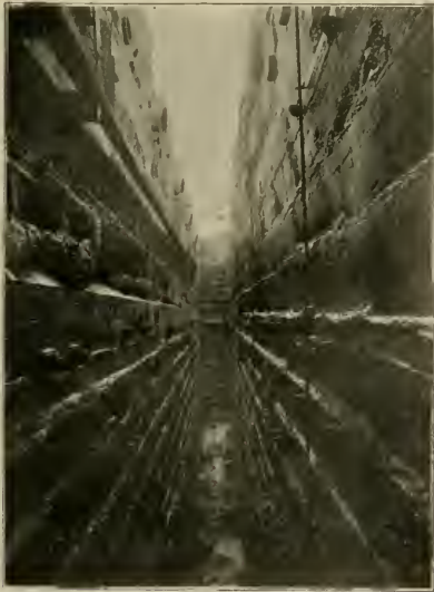
THE NEW WHEEL PIT.
