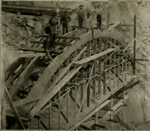
FALSE WORK FOR ARCHES.
