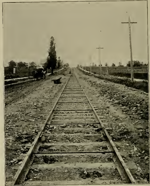
SIX INCH 60-LB. T RAIL, OAKLAND AVENUE, MILWAUKEE.
