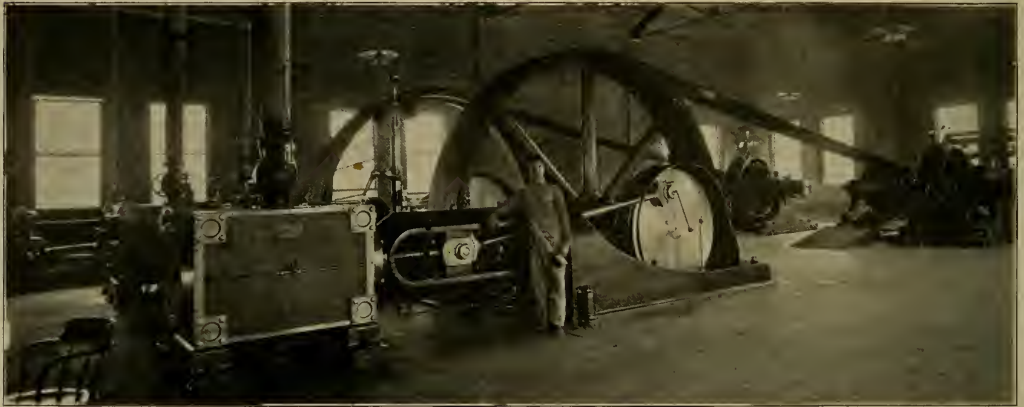
INTERIOR OF CUYAHOGA FALLS POWER HOUSE—A., B. & C. R. R.
