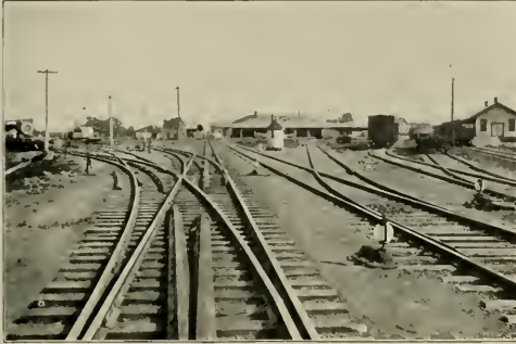
THIRD RAIL AT SWITCH.
