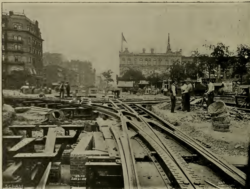
CURVE AND CROSSINGS AT FIFTY NINTH STREET AND EIGHTH AVENUE.
