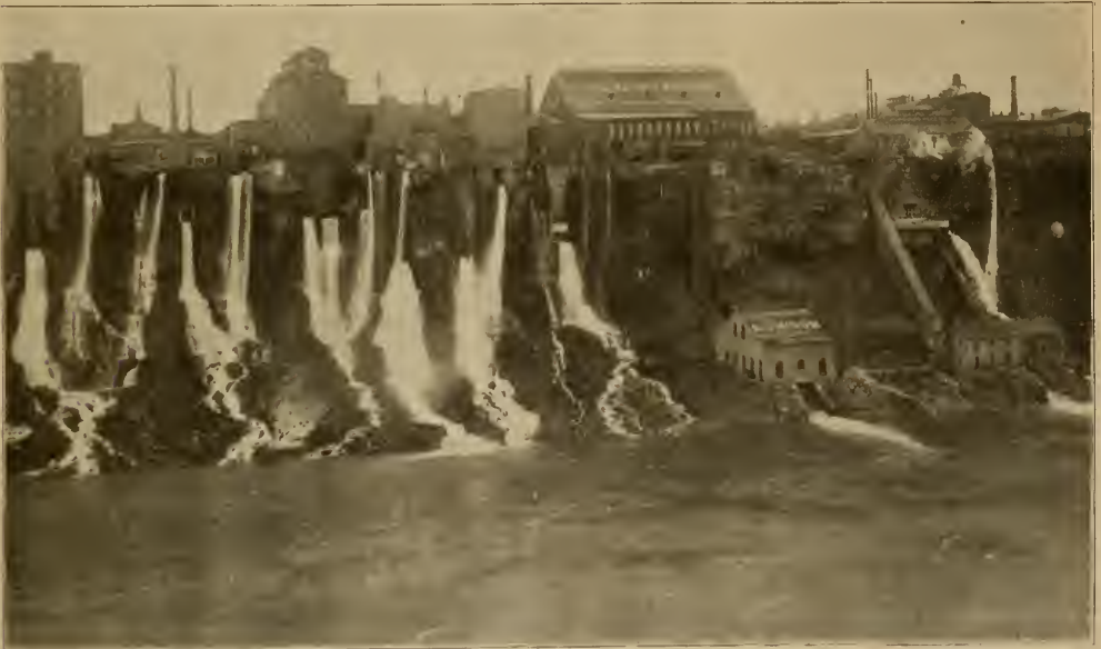
NIAGARA FALLS HYDRAULIC POWER AND MANUFACTURING COMPANY.
