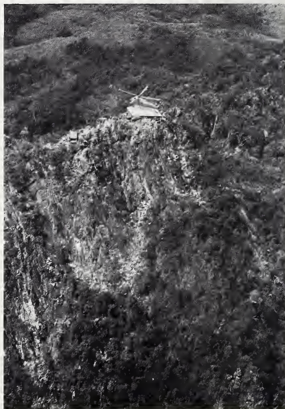
Department of Defense Photo (USMC) A188645 A UH-34D from Marine Medium Helicopter Squadron 163 uses a newly constructed helicopter pad on top of the Rockpile to resupply members of the 3d Battalion, 3d Marines. Helicopters previously performed this mission by hovering with one wheel on a tiny wooden ramp. (See photograph on page 183 of the volume U.S. Marines in Vietnam, 1966.)
