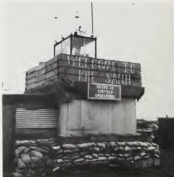
Department of Defense Photo (USMC) A189984 Men from Marine Air Traffic Control Unit 62, a subordinate unit of MAG-12, operate at the Khe Sanh airstrip from expeditionary equipment they have sandbagged against NVA artillery and rockets.
