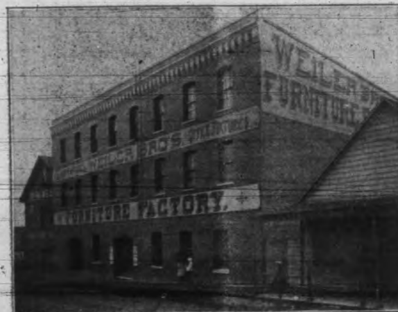
FURNITURE FACTORY, Humbolt Street, foot of Douglas. The finest store, bank, saloon and office fixtures in Victoria and adjacent cities are manufactured here.
