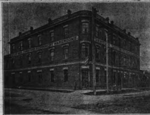
WAREROOMS, corner of Broughton and Broad Streets; Rambler Cycles in corner.
