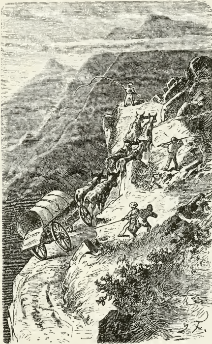
WAGGON-ROAD OVER THE DRAKENBERG.
