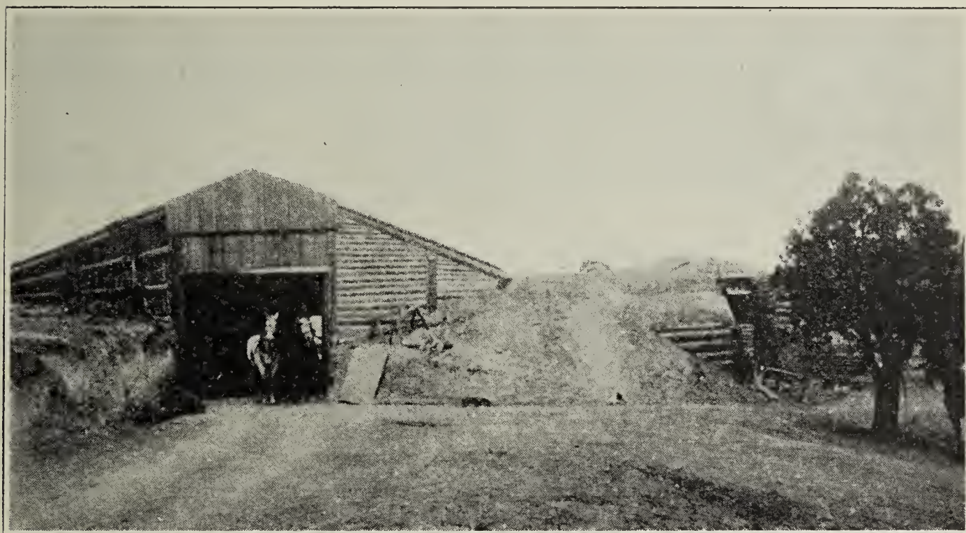
An Up-to-date Potato Cellar; Capacity 25,000 bushels; at Carbondale, Colorado.
