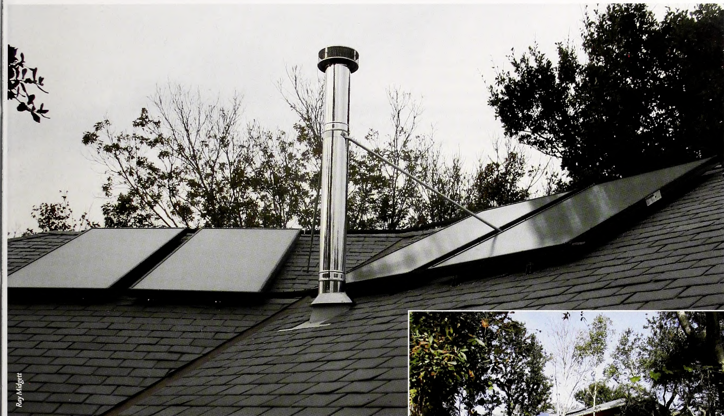
ABOVE: South-facing solar panels collect energy from the sun. Roofing shingles look like slate, but are made from recycled rubber and plastic materials. RIGHT: The Arizona-style home is nestled among live oak trees.
