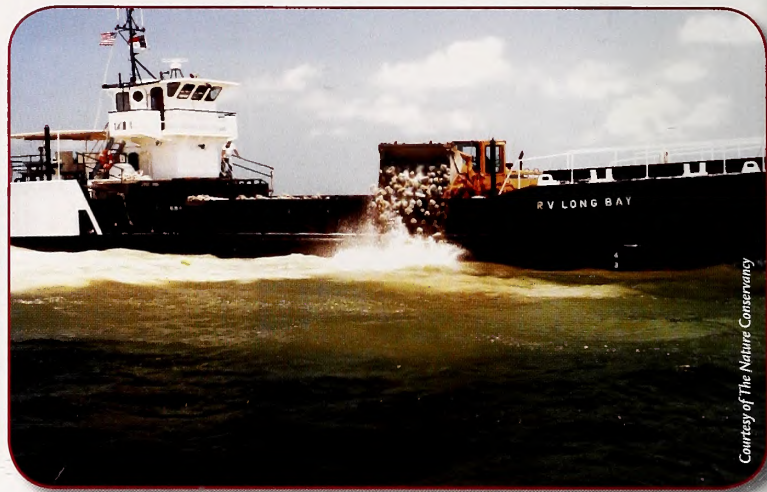
LEFT: BALLANCE'S WORK HAS HELPED IMPROVE THE SITE SELECTION PROCESS FOR OYSTER RESTORATION. RIGHT: A BARGE EMPTIES SEVERAL HUNDRED TONS OF LIMESTONE MARL TO CREATE A RESTORATION SITE.
