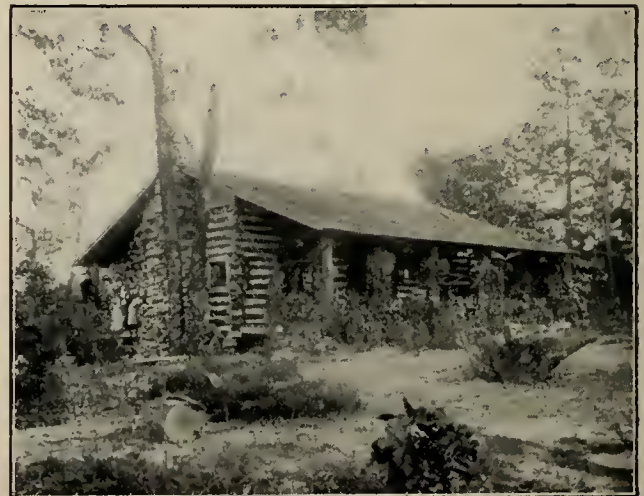
COTTAGE (ERECTED BY MRS. E. E. HOSS) ON BROW OF MOUNTAIN.
