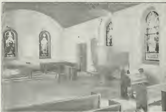
INTERIOR VIEW OF THE CHURCH, 1907.
