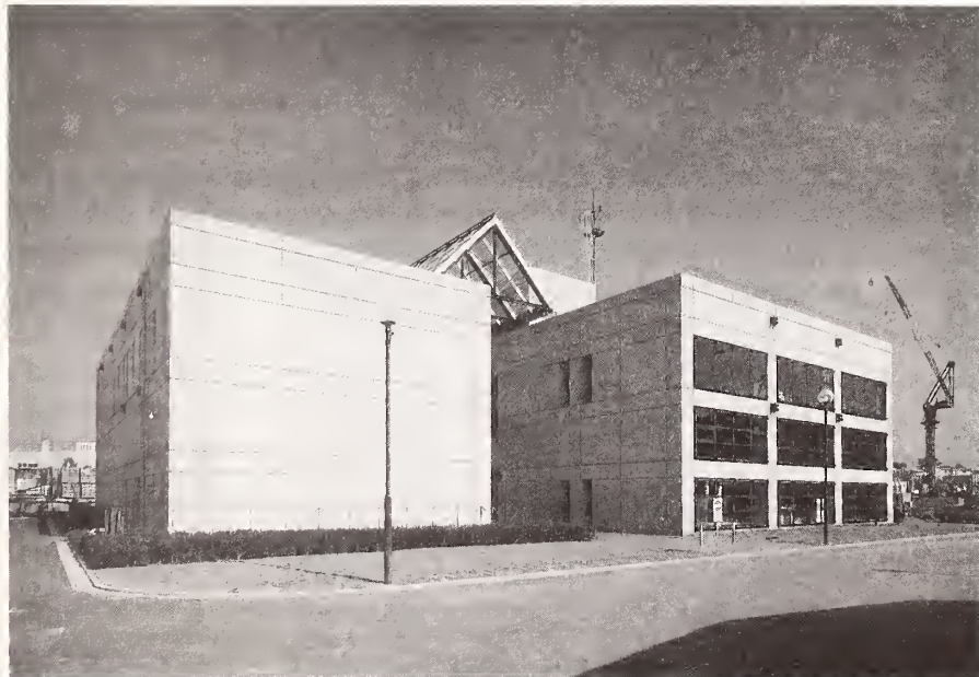
View of the acoustic and environmental vibration test building. (Left - base isolation building; Right - building with conventional technique).
