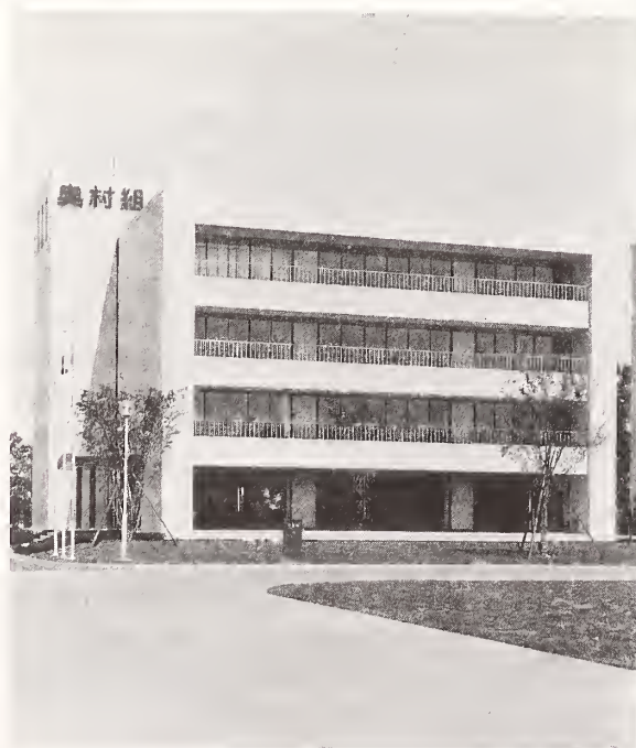
View of the administrative wing
