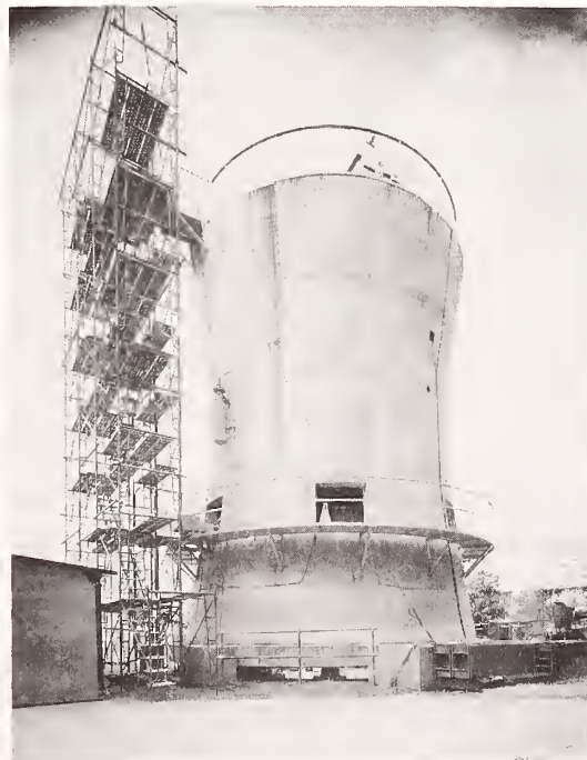
Large-scale experimental structure
