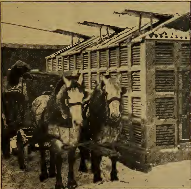
Being fire-proof, rat-proof, and permanent are the merits of this hollow-tile cornerib. It will last for years without repairs
