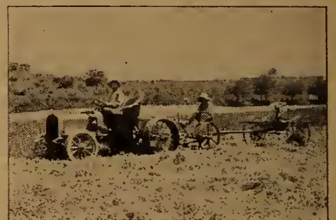
The tractor could pull the tedder as well as the mower, so two operations were performed at once. Slow to very fast speeds were used. When the weather was hot, or when work was pressing, we used the lighting system and worked at night. Corners were turned round
