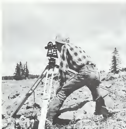
Engineers surveying for a new road in Grand Mesa National Forest, Colorado. The layout of this road was done from aerial photographs using the latest photogrammetric techniques.
