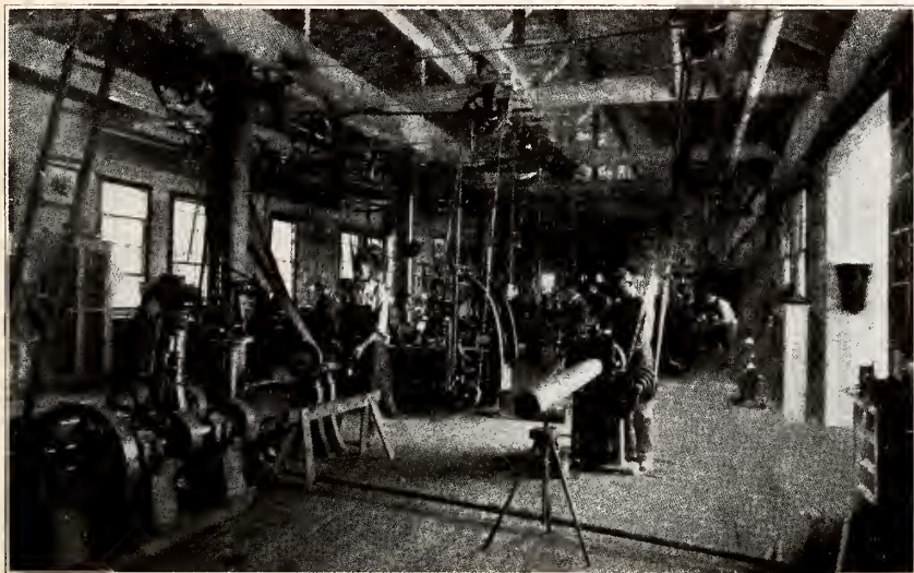
A CORNER IN THE MACHINE SHOP.
