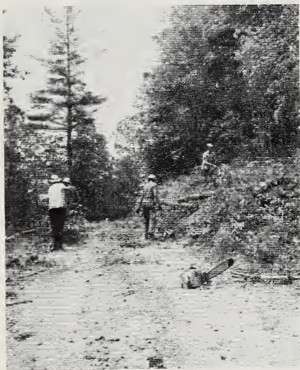
The road to Scotchman Creek. It cost Haywood EMC $8,500 to build a line through this remote territory in order to bring electric power to Mr. McCall.
