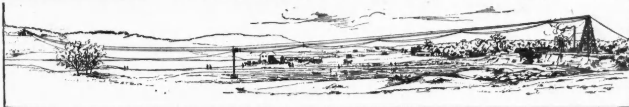
LIDGERWOOD CABLEWAY, AUSTIN DAM—1,350 feet span.
