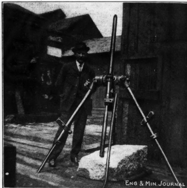
THE FOLLOW-UP DRILL MOUNTED ON A TRIPOD
