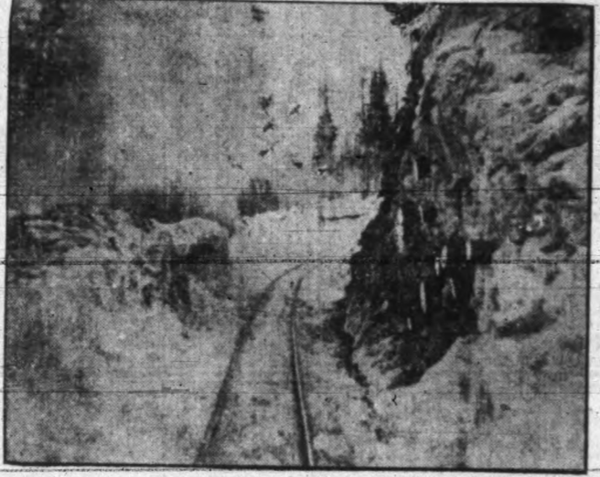
SCENE IN ROGER'S PASS. Cutting Made Through Previous Slide, Showing Trees Carried Down With Debris.
