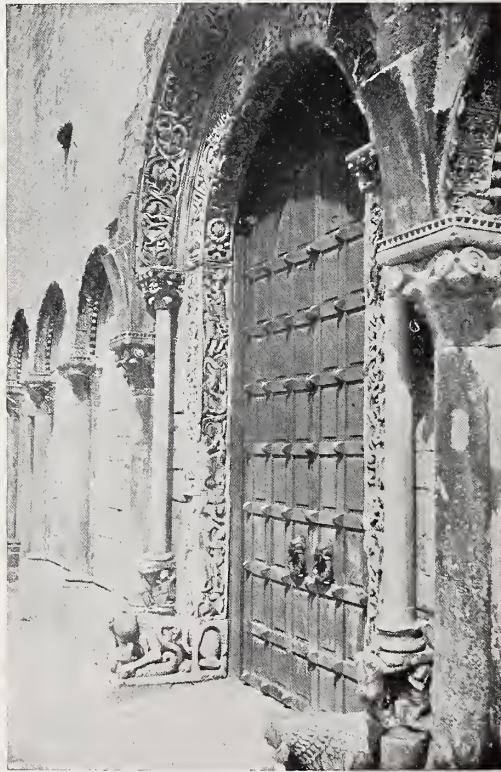
Fig. 217.—Trani, Cath., Doorway.
