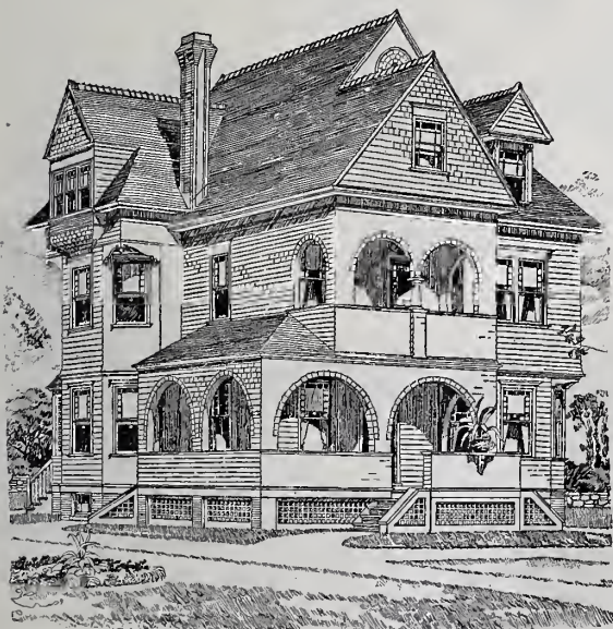
A Builder's Design.—Example of crude work.
