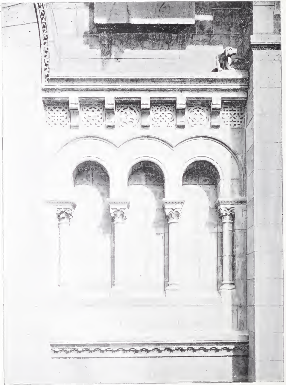
ARCADE ON WEST FAÇADE.
