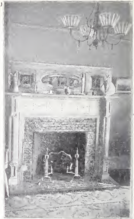
Mantelpiece by W. S. Knowles, Architect.
