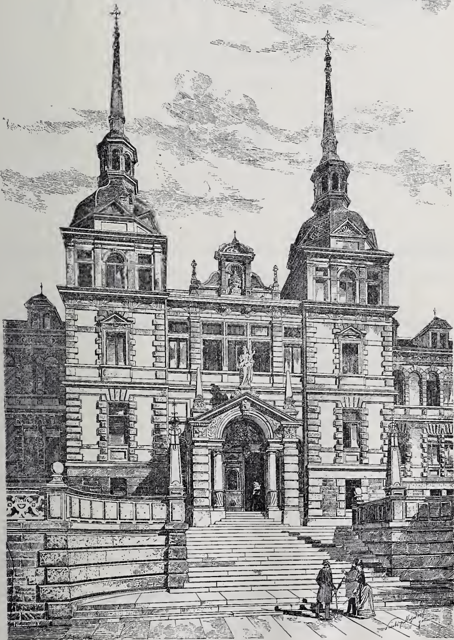
MIDDLE BUILDING OF ST. MARY'S HOSPITAL.
