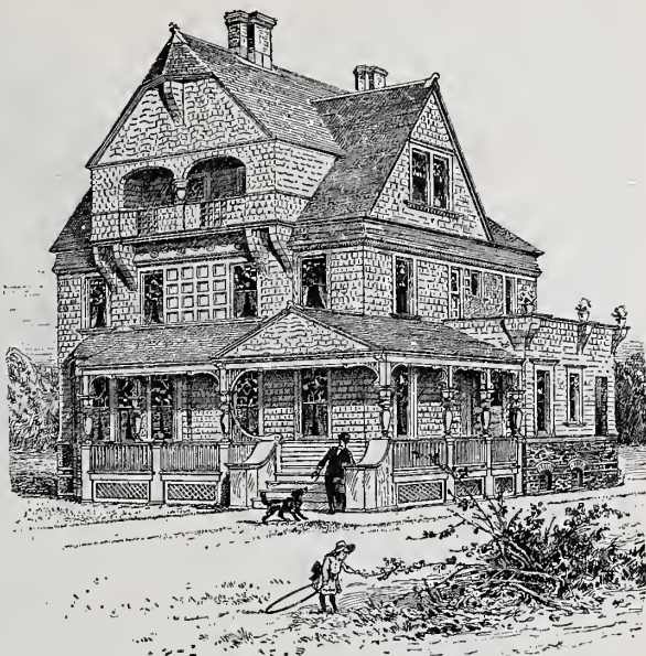
A Builder's Design.—Example of crude work.
