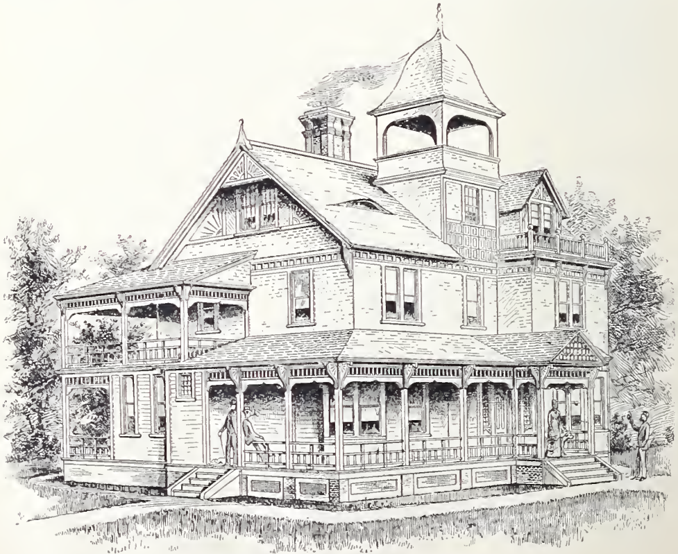
A Builder's Design.—Example of crude work.
