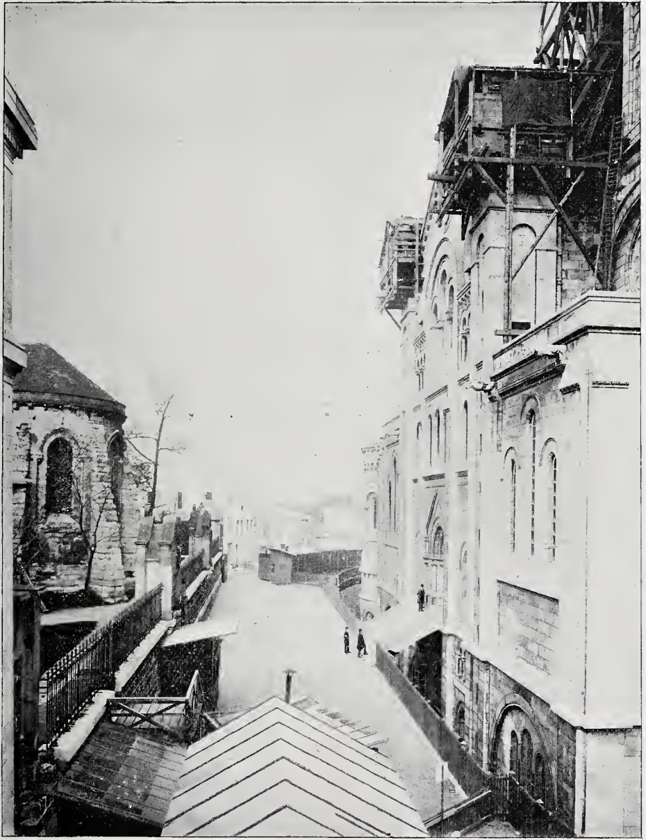
VIEW OF WEST FAÇADE.
