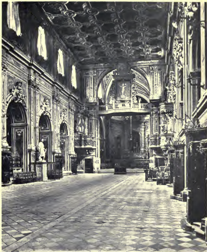
Fig. 41.—Naples. Church of the Carmine. Interior.
