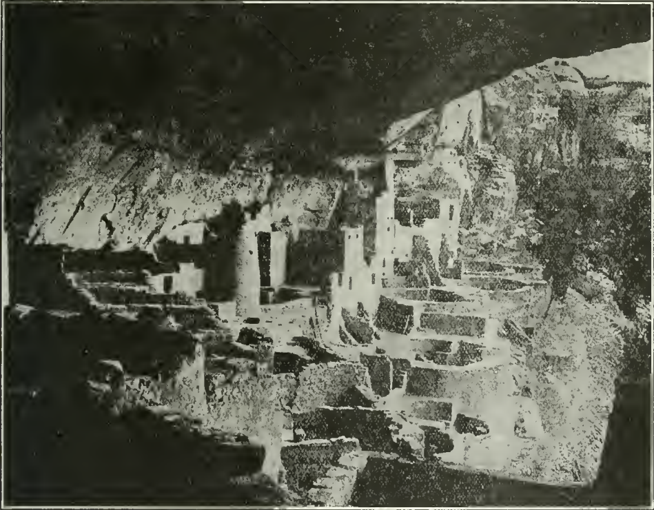
Photograph, Department of Interior
