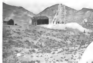
Hoisting Works at the New York Tonopah Mine
