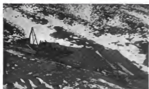
Top Workings at the Ray Mine
