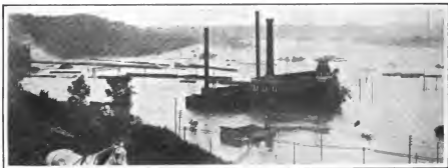
The Turkey Creek Pumping-Station, which is the only Source of Water Supply for Kansas City. The Station was of course ruined
