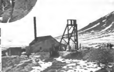
Power Plant and Hoist at the Halpax
