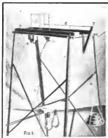
Diagram of the Albertson Magnetic Train, showing the Force required to move an empty Car
