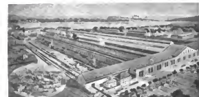
Plant of Riser-Conley Manufacturing Company, Pittsburgh, Pennsylvania
