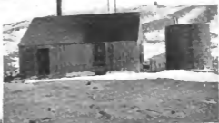
Pumping Station which supplies Tonopah with Water
