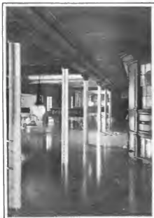
Interior of the Union Station, Kansas City, with Three Feet of Water above the Floor
