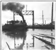
Relief Trains at the Crossing of Missouri Avenue. The Tracks are entirely under Water
