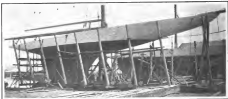
"Reliance" in Dry Dock, showing the extraordinary Overhanging Mast
