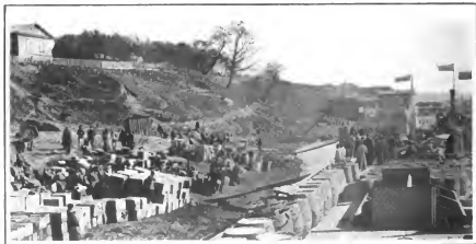
Building the Town of Harbin, in Central Manchuria, with Materials sent from America
