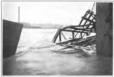
Wreck of the Elevated Railway where it crosses the Kansas River The great force of the Flood is shown clearly in the Photograph
