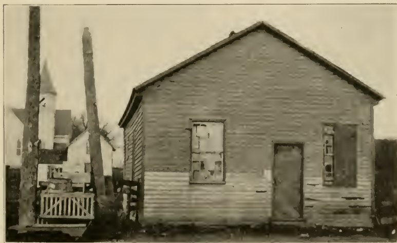
OLD SCHOOLHOUSE, NEW CALIFORNIA. (Erected 1852.)
