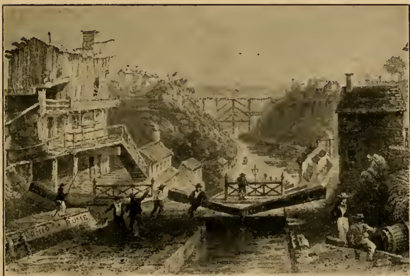
THE LOCKS AT LOCKPORT ON THE ERIE CANAL
