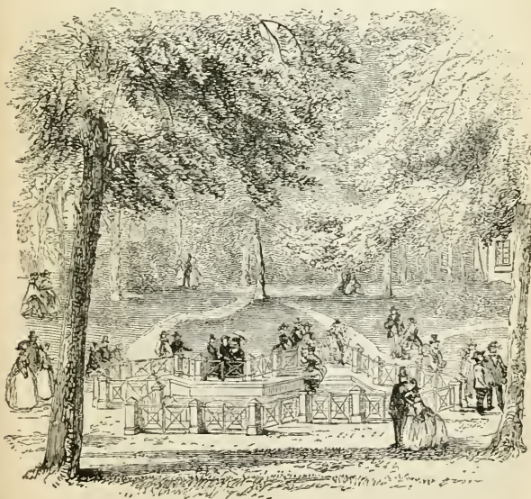
THE STAHL-BRUNNEN (STEEL WELL) IN THE KUR-GARTEN.
