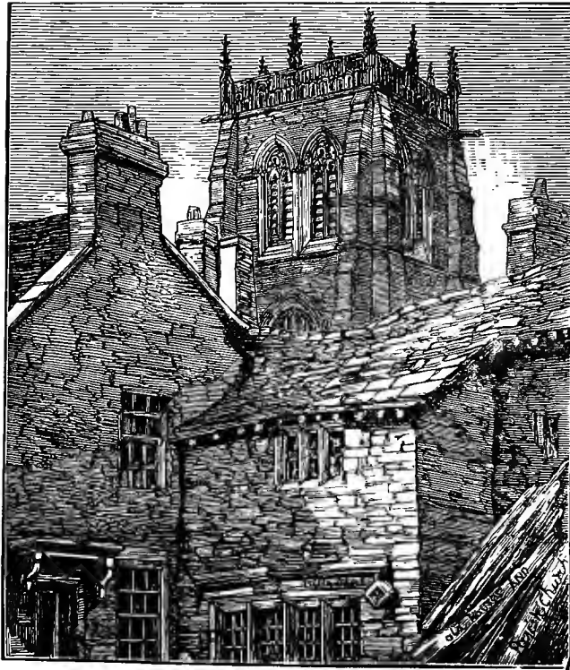
Old Houses and Parish Church.
