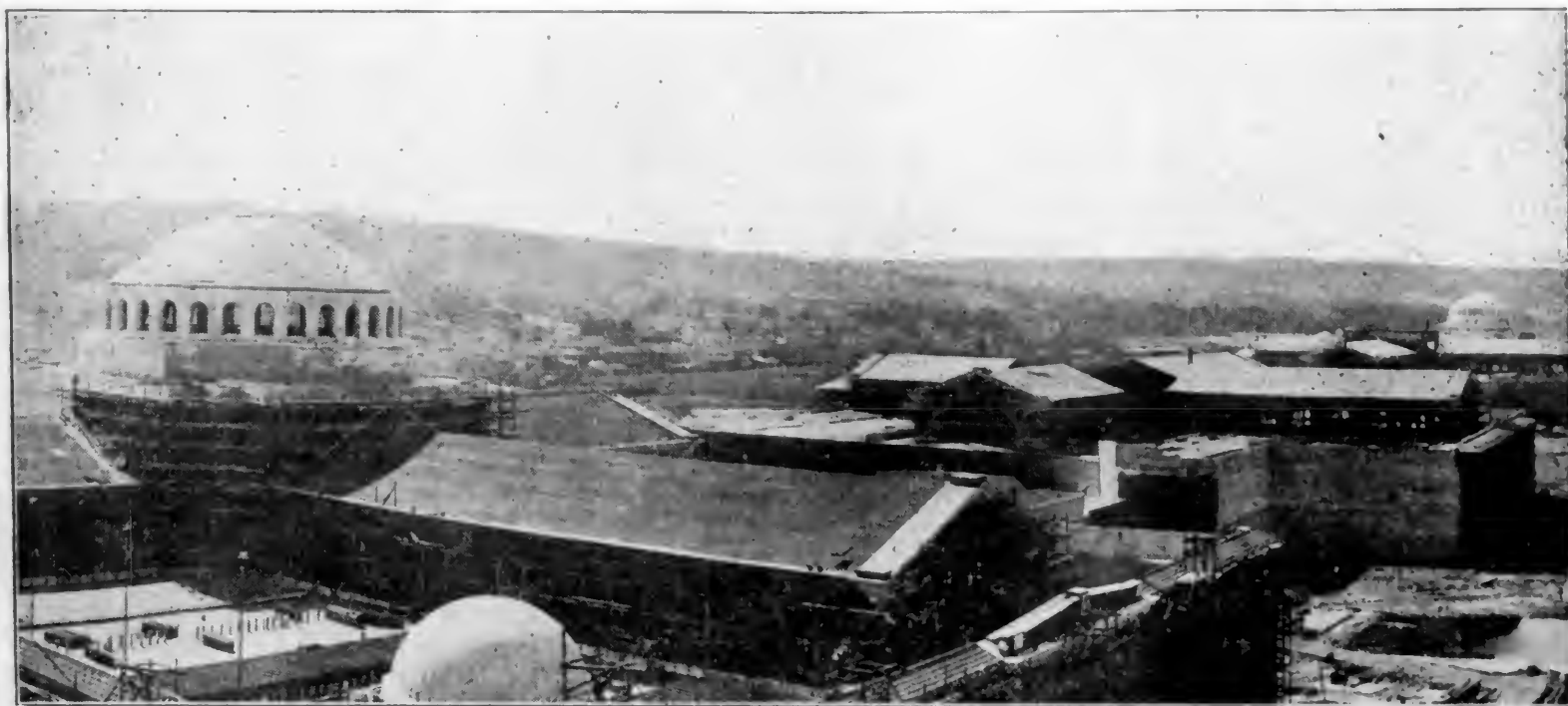
The panoramic photograph taken from the top of the Palace of Machinery March 1st, shows the remarkable progress of the construction of the Panama-Pacific International Exposition. The Palace of Machinery has been the left is the Palace of Varied Industries, and in its rear the Palaces of Manufactures, Liberal Arts and the Court of the Universe, in which will be sunken garden capable of seating ten thousand people; to the rear of that the Court of Four Seasons, and directly behind that same distance will be the Palace of Fine Arts.
