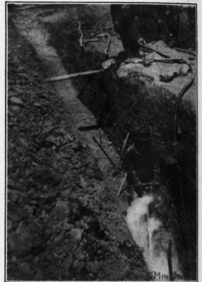
TRENCHING WITH STEAM PLUG DRILL
