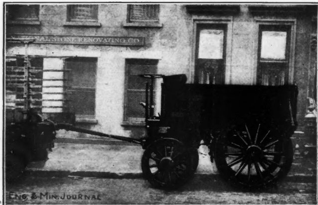
FIVE-TON TRAILER FOR MCCONNELL MINE
