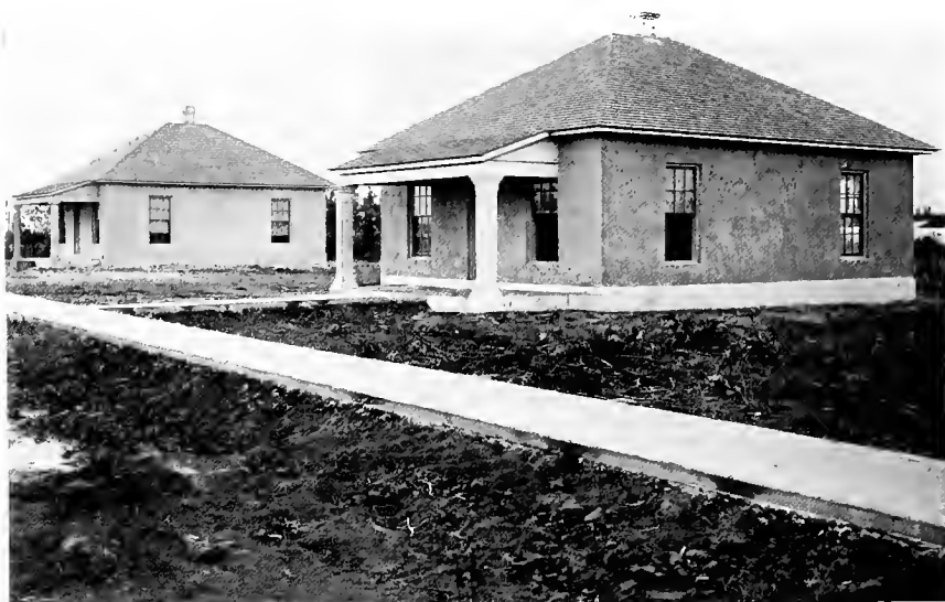
Fig. 2.—One-story concrete workingman's cottage, exemplifying simple and direct use of concrete.
