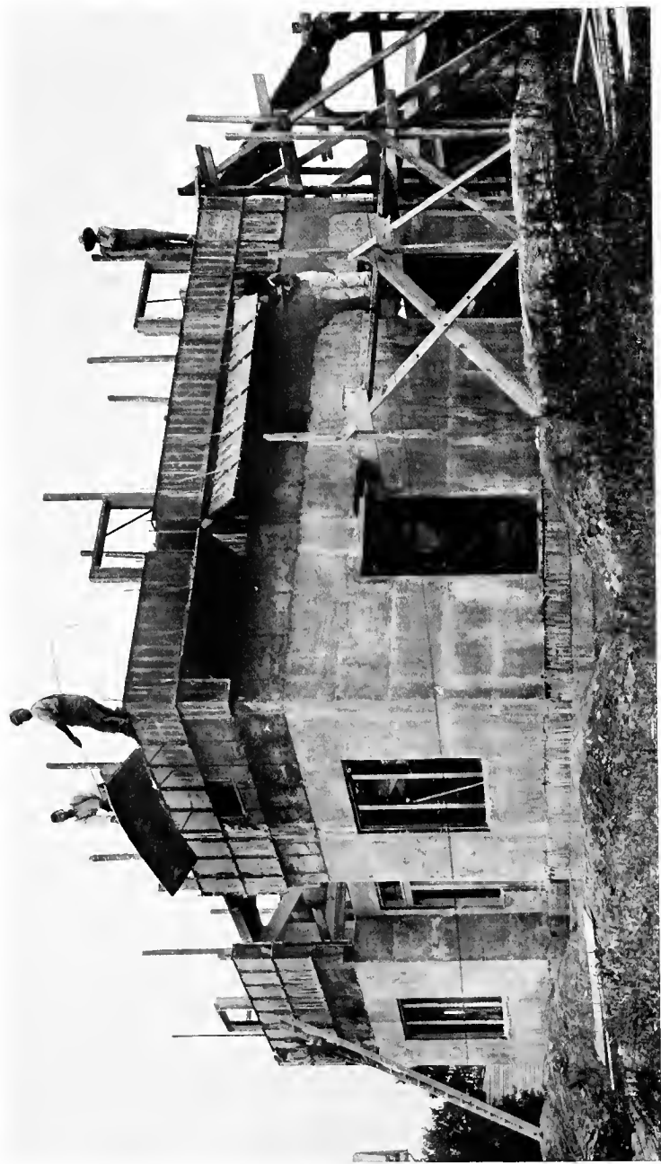
Method of raising and adjusting steel forms by the two-tier process. Forms designed and patented by Read & Morrill, Brooklyn, N. Y.
