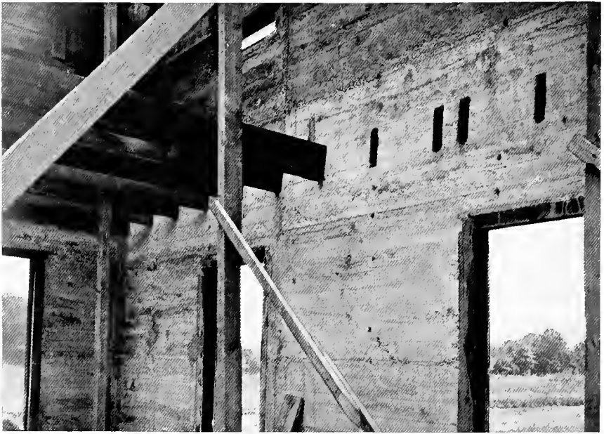
Wall recesses for timber joist.
