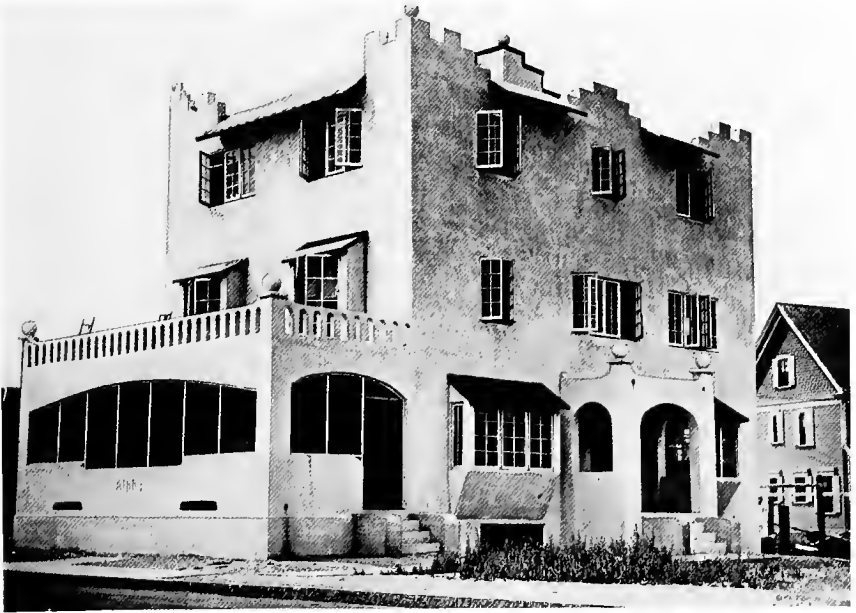
Fig. 7.—A porch illustrating the practicability of long span construction in concrete.
