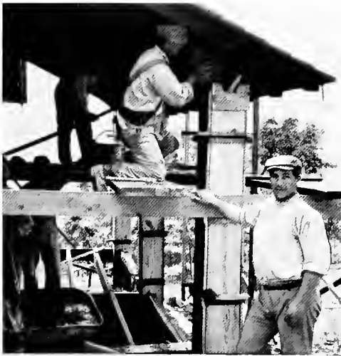
Pouring concrete into a column form.
