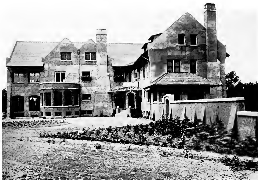
Fig. 3.—A carefully studied design, showing frank treatment of concrete walls and surface finish.
