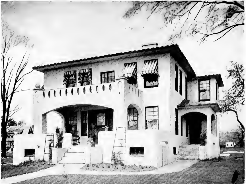
Fig. 10.—A second example of the adaptability of concrete to long span construction. Note porch.
