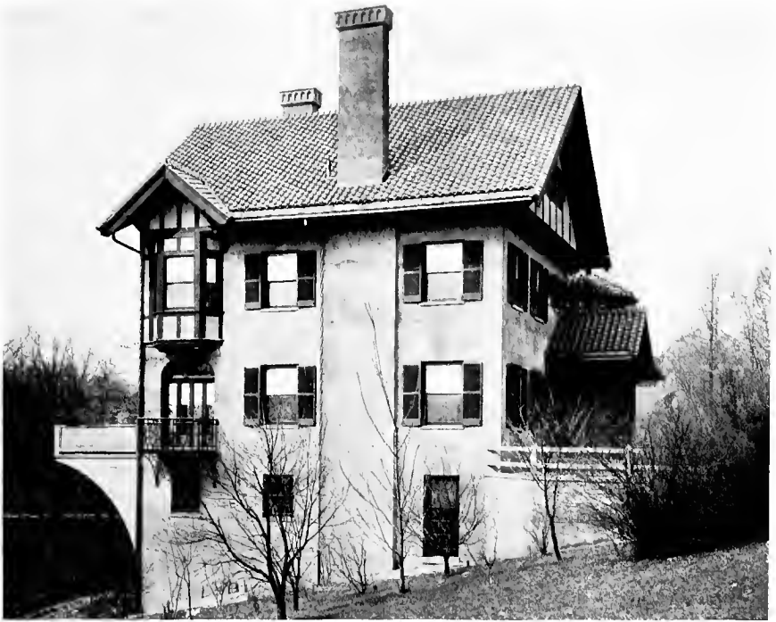
Fig. 5.—A house showing the adaptability of concrete to the construction of projecting masonry.
