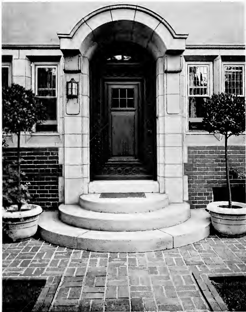
Entrance of Albert Kahn's residence, Detroit, Mich. Doorway and steps cast in solid concrete. A striking example of the economy of concrete as compared with cut stone.
