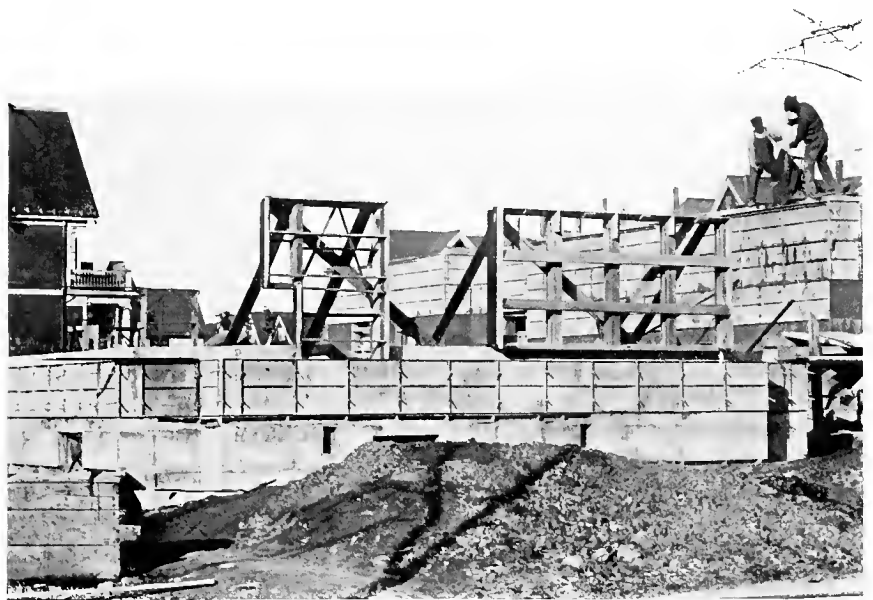
Patented steel forms in use.
