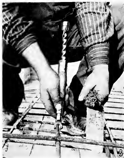
Fig. 77.—“Curry Tyer.” A convenient method for wiring reinforcement together.
