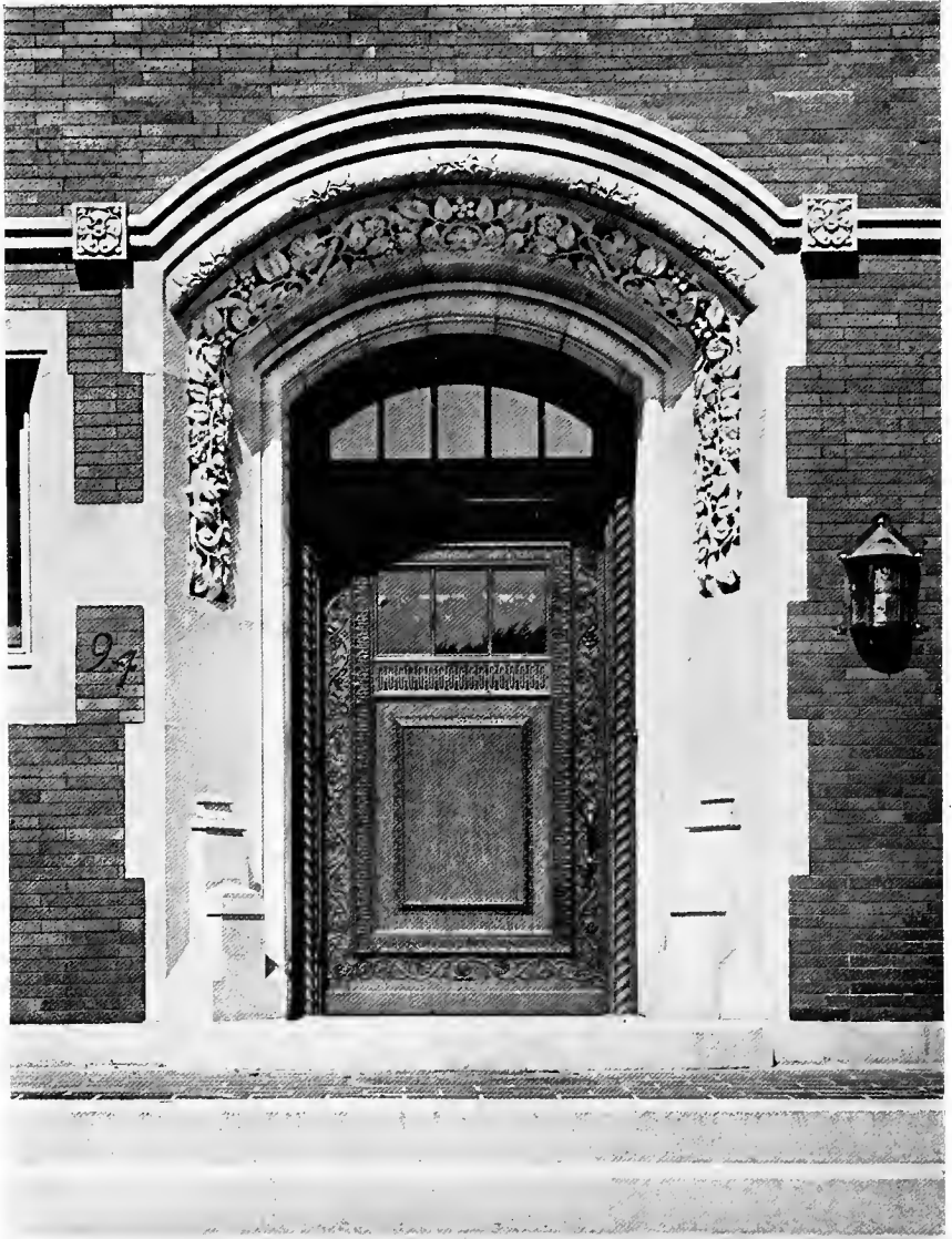
A doorway showing the adaptability of concrete to either plain or ornamental work. Note the great contrast between the elaborate undercut floral decoration and the simple units comprising the structural features.
