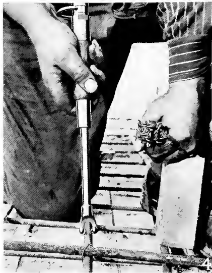
Fig. 77.—“Curry Tyer.” A convenient method for wiring reinforcement together.
