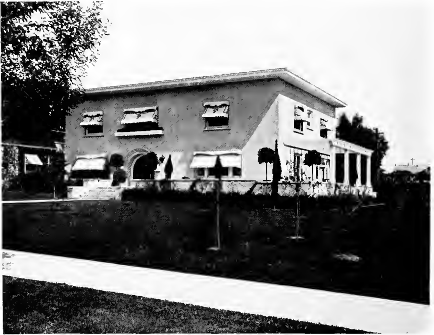
Fig. 8.—A beautiful house in which concrete has been consistently treated throughout.
