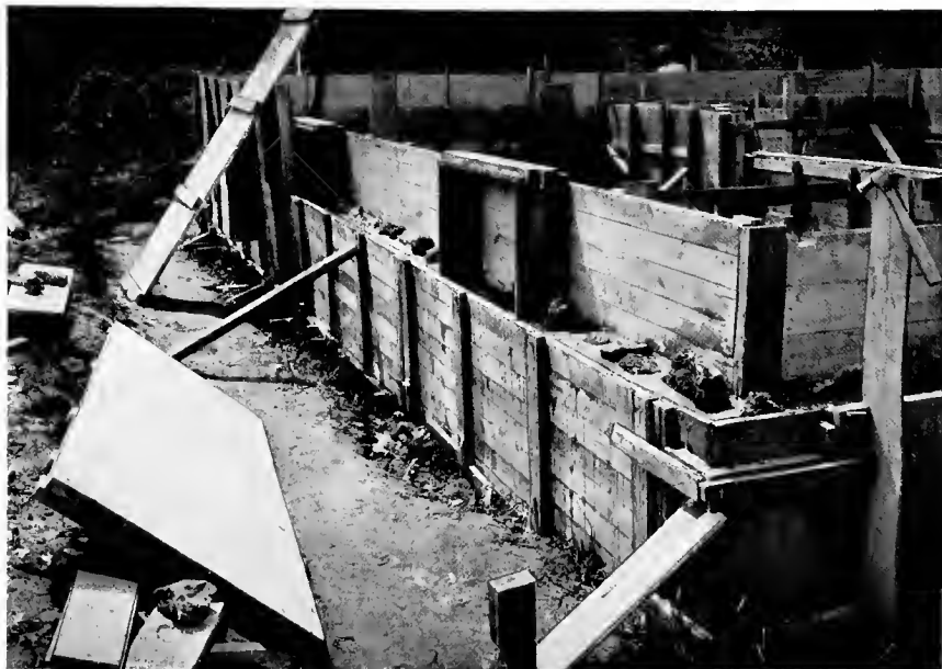
Typical sectional form for concrete wall construction.
