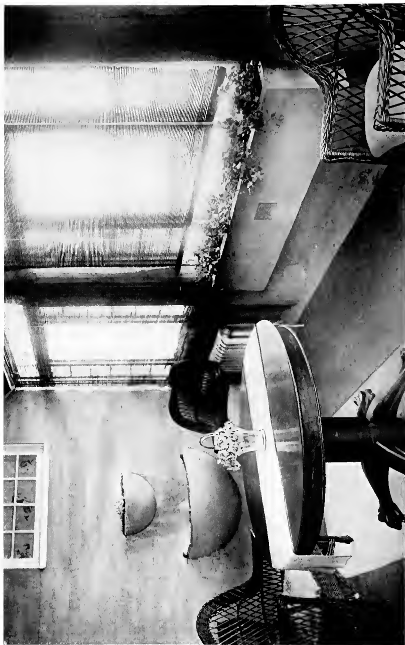
A concrete living room porch in a seashore house. Note concrete flower boxes anchored to the walls and fountain cast with concrete partition. Dampness has never penetrated partition wall.
