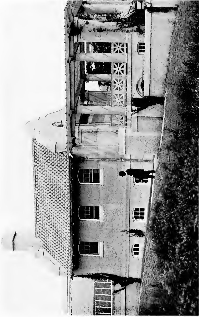
A dwelling showing adaptability of concrete to varied details of construction. It is used here for walls, chimney, columns, balustrade and floors. Aberthaw Construction Co., Boston
