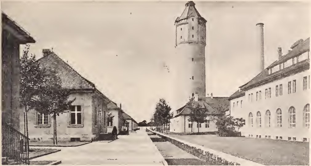
WATER TOWER AND ELECTRICAL PLANT.
