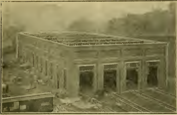
VIEW OF THE EXTERIOR OF THE PAINT SHOP BUILDING. (TAKEN FROM ROOF OF ERECTING SHOP.)
