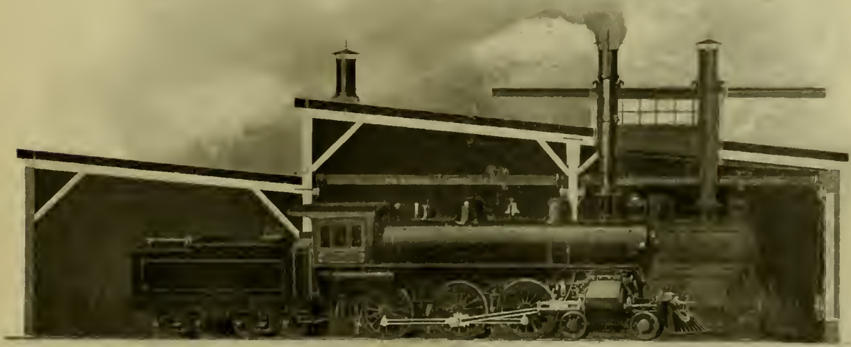
ROUNDHOUSE EQUIPPED WITH OVERHEAD CRANES AND MOVABLE TELESCOPIC SMOKE JACKS.
