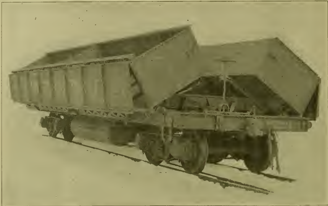
LAWSON DUMP CAR WITH BOTH BOXES IN DUMPED POSITION.
