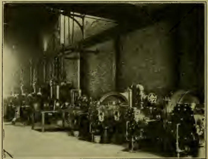
ENGINE ROOM VIEW, SHOWING STEAM PIPING ARRANGEMENT. RAND AIR COMPRESSORS AT RIGHT.
