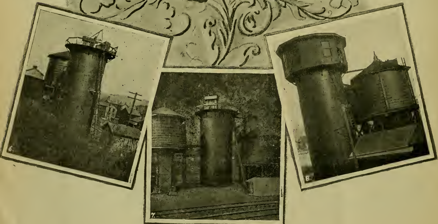
THE 42,000-GALLON PLANTS AT (1) STOBO, PA.; (2) NEW CASTLE JUNCTION, PA.; (3) HAZLETON, O.; (4) ROCK POINT, PA., AND (5) GROVETON, PA. THE 21,000-GALLON PLANTS AT (6) WILLIAMSBURG, PA.; (7) WHITSETT JUNCTION, PA., AND (8) BUENA VISTA, PA. VIEWS OF REPRESENTATIVE INSTALLATIONS OF THE WATER-SOFTENING SYSTEM.—PITTSBURG & LAKE ERIE RAILROAD.
