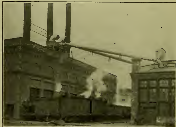
VIEW OF THE EXHAUSTER LEADS DELIVERING SHAVINGS FROM THE CABINET SHOP AND WOOD MILL TO THE BOILER ROOM STORAGE BINS.
