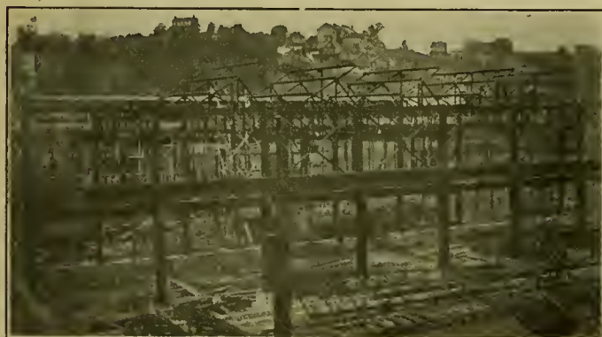
CONSTRUCTION VIEW OF THE BOILER SHOP BUILDING.
