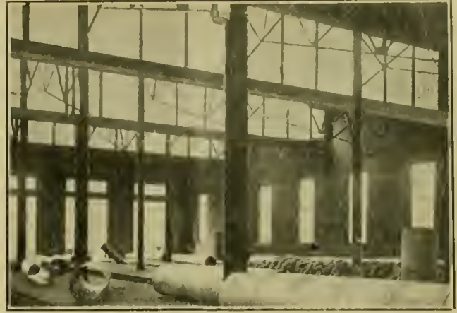
INTERIOR VIEW OF PAINT SHOP, SHOWING PROFUSE CHARACTER OF THE DAYLIGHT LIGHTING FROM THE SAW-TOOTH SKYLIGHTS.
