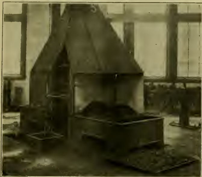
FIG. 3.—CAST IRON DOUBLE FORGES.
