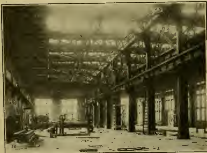
INTERIOR VIEW OF THE BOILER AND TANK SHOP, IN BOILER MACHINE BAY. (LOOKING NORTH.)
