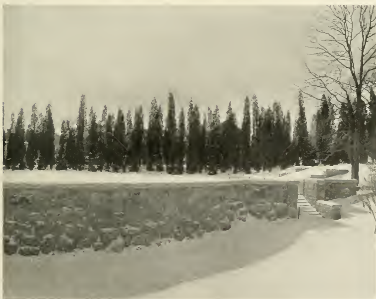
PLAZA AT BOSTON ROAD ENTRANCE. View Directly South, After Planting and Terrace Wall were Completed.
