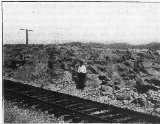
Fig. 3—Railroad cut in Sec. 32, T. 23 S., R. 60 E., showing location of joints that bear carnotite
