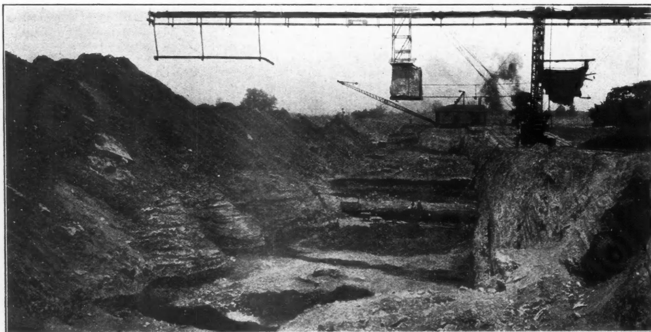
Hoover & Mason mine, showing cantilever in foreground and drag-line in distance
