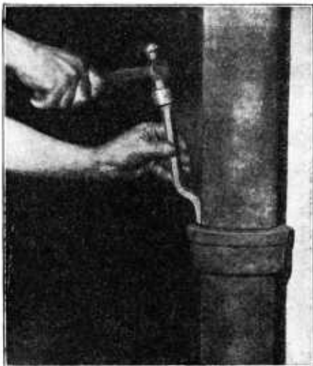
FIGURE 8.—Calking a lead joint to make it air-tight and water-tight.
