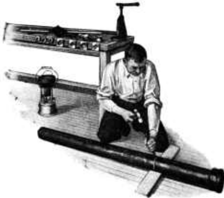
FIGURE 6.—Cutting cast-iron pipe with a cold chisel.
