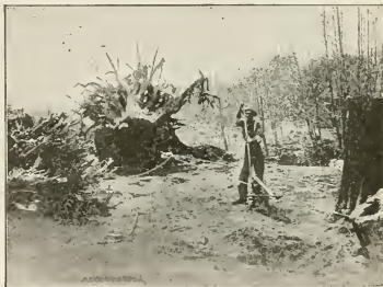
THE "K" POWER PULLER AT WORK.
