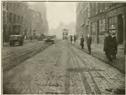
RUBBER PAVING IN BOROUGH HIGH STREET, SOUTHWARK.
