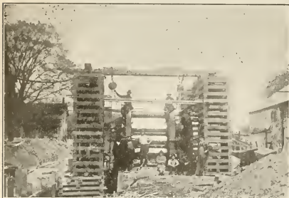
IN ORDER TO SAVE TIME AND TO COMMENCE PRODUCTION AT THE EARLIEST POSSIBLE DATE IN HIS NEW PLANT AN ENTERPRISING RUBBER MANUFACTURER IN THE AKRON DISTRICT INSTALLED THE CALENDER BEFORE THE BUILDING WAS ERECTED.
