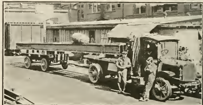
OCASIONS SOMETIMES ARISE WHEN TRUCK OVERLOADING IS UNAVOIDABLE. IN SUCH CASES, SOLID TIRES PROVE THEIR WORTH. THE TRUCK SHOWN ABOVE CARRIES 22,000 POUNDS OF STEEL BEAMS. THE LOAD WAS BROUGHT OVER BAD STRETCHES OF ROAD BETWEEN PITTSBURGH AND AKRON WITHOUT MISAP.
