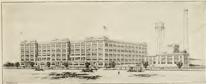
NEW PLANT OF THE SEAMLESS RUBBER COMPANY, INC., NEW HAVEN, CONNECTICUT.
