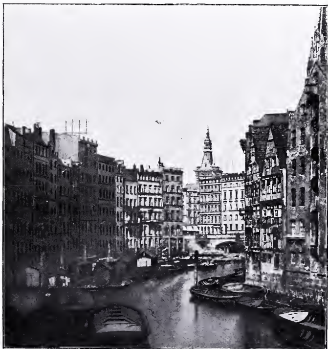
FLEET DEICHSTRASSE IN HAMBURG
