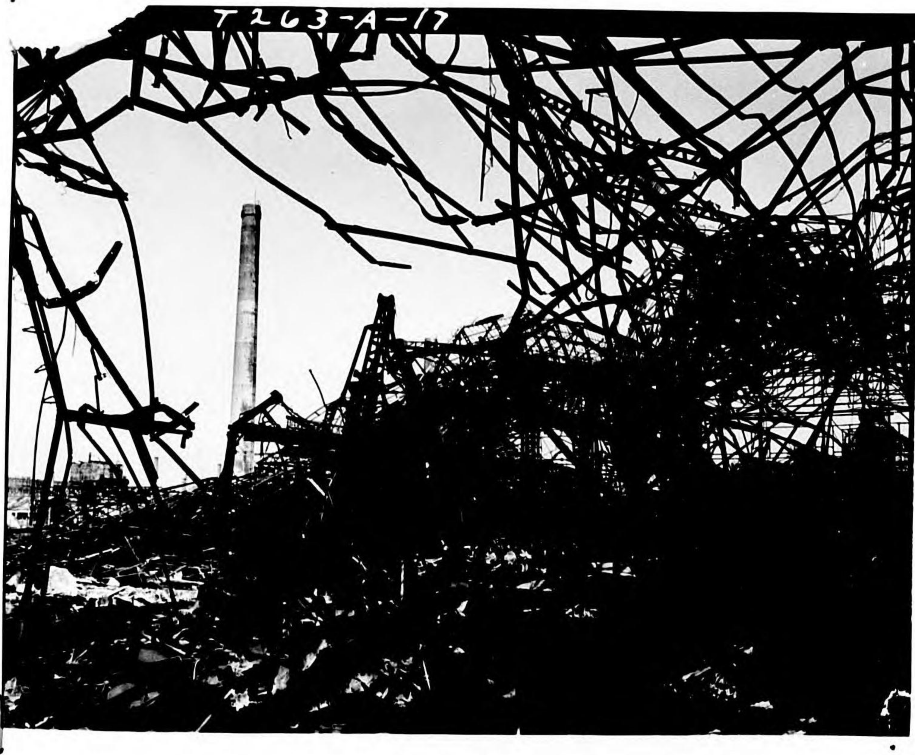
Photo 18 - Bldg. 51, Bomb 90. Structural failure roof and columns.
