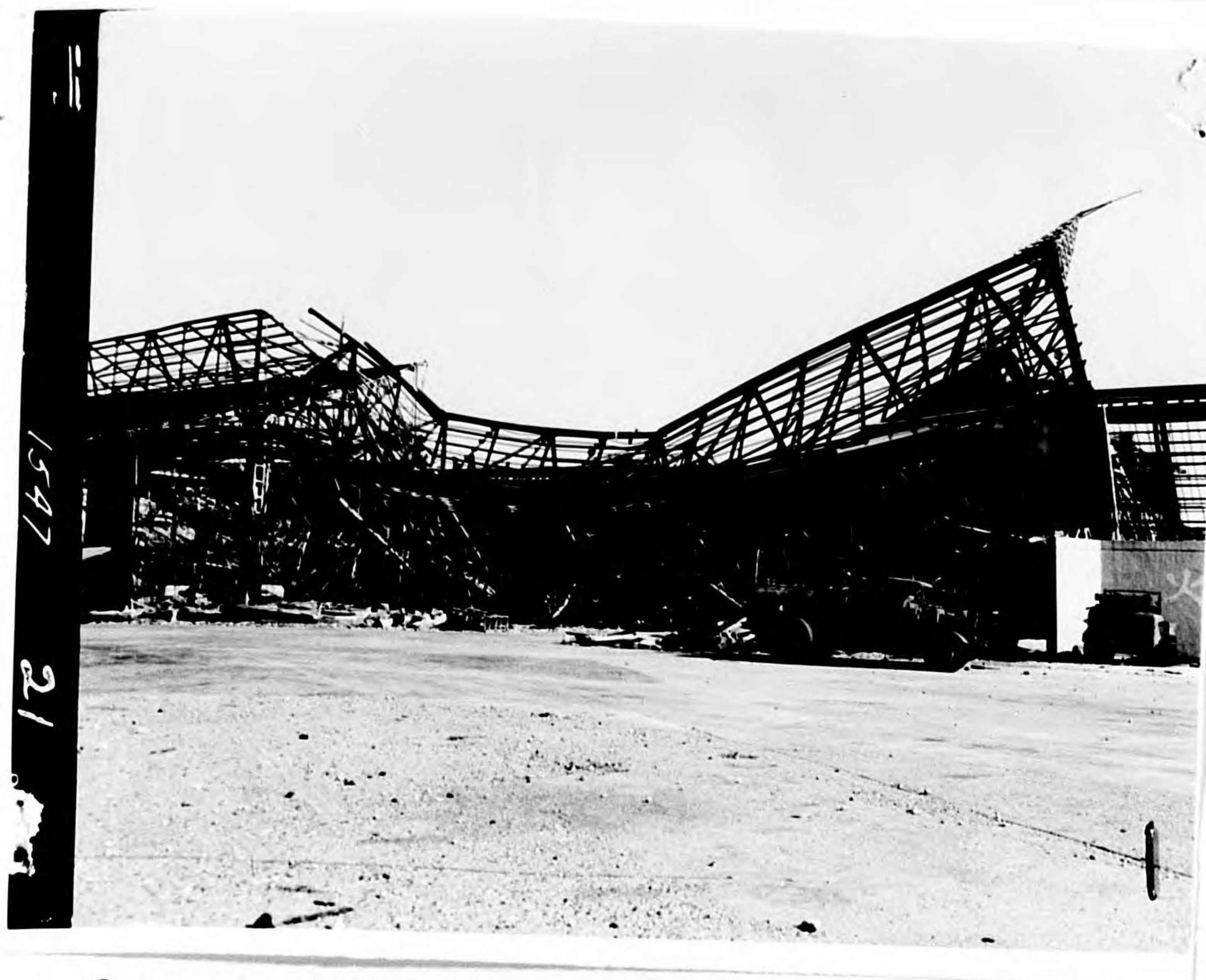
Photo 21 - Bldg 22, Bomb 3, General view of Collapse.
