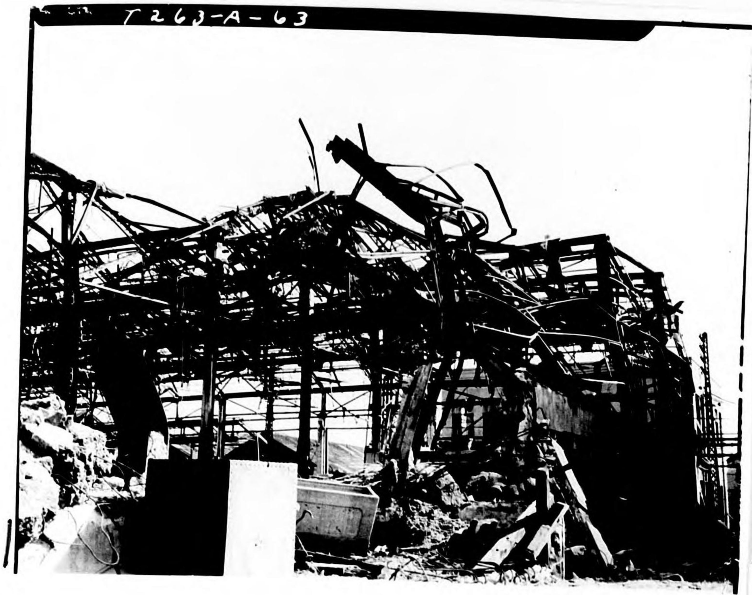
Photo 1 - Bldg. 3. Bomb 42. Blasted bent and folded columns.
