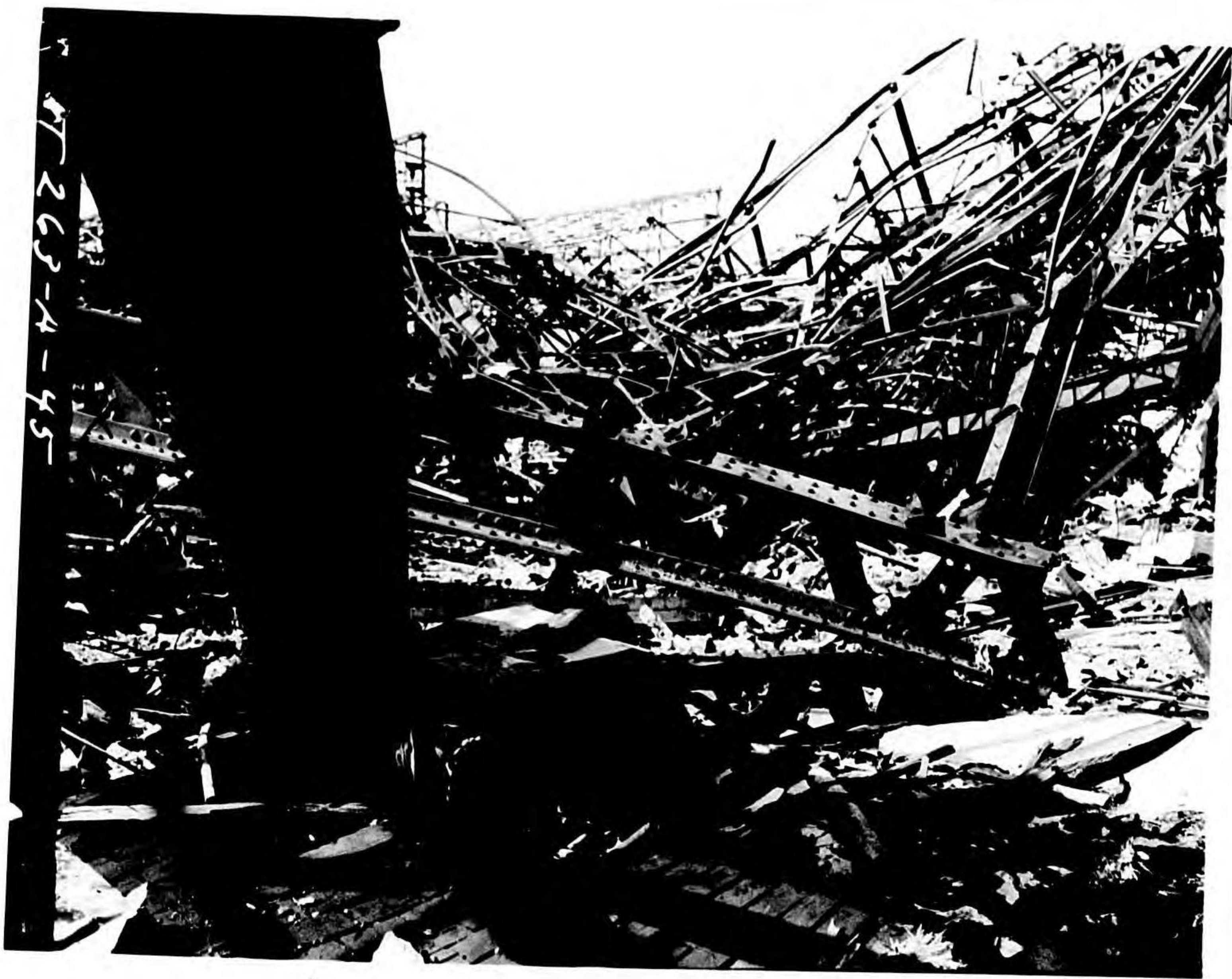
Photo 16 - Bldg. 51, Bomb 66. Detail of column damaged.
