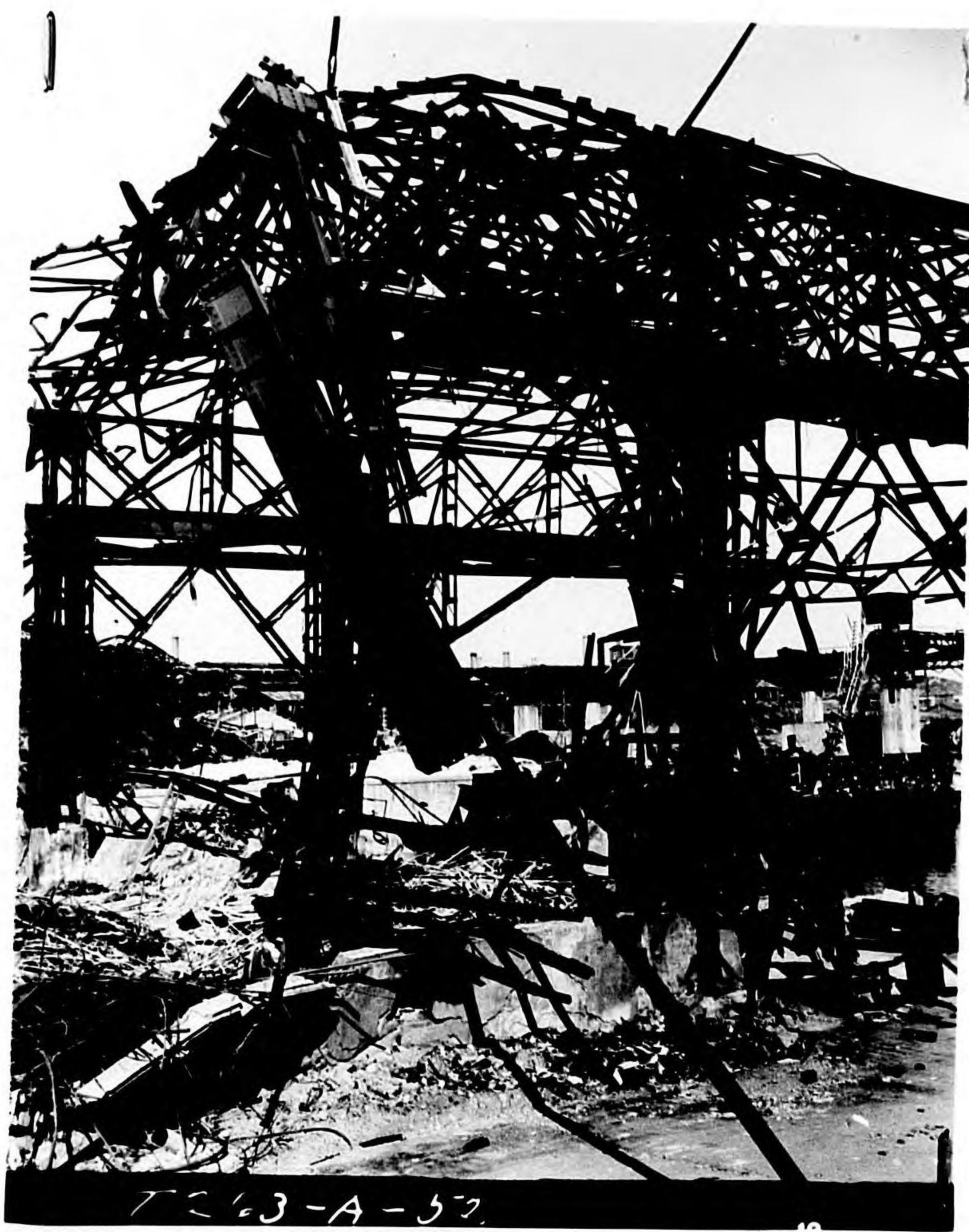
Photo 8 - Bldg. 33, Bomb 71. Roof damage from column.
