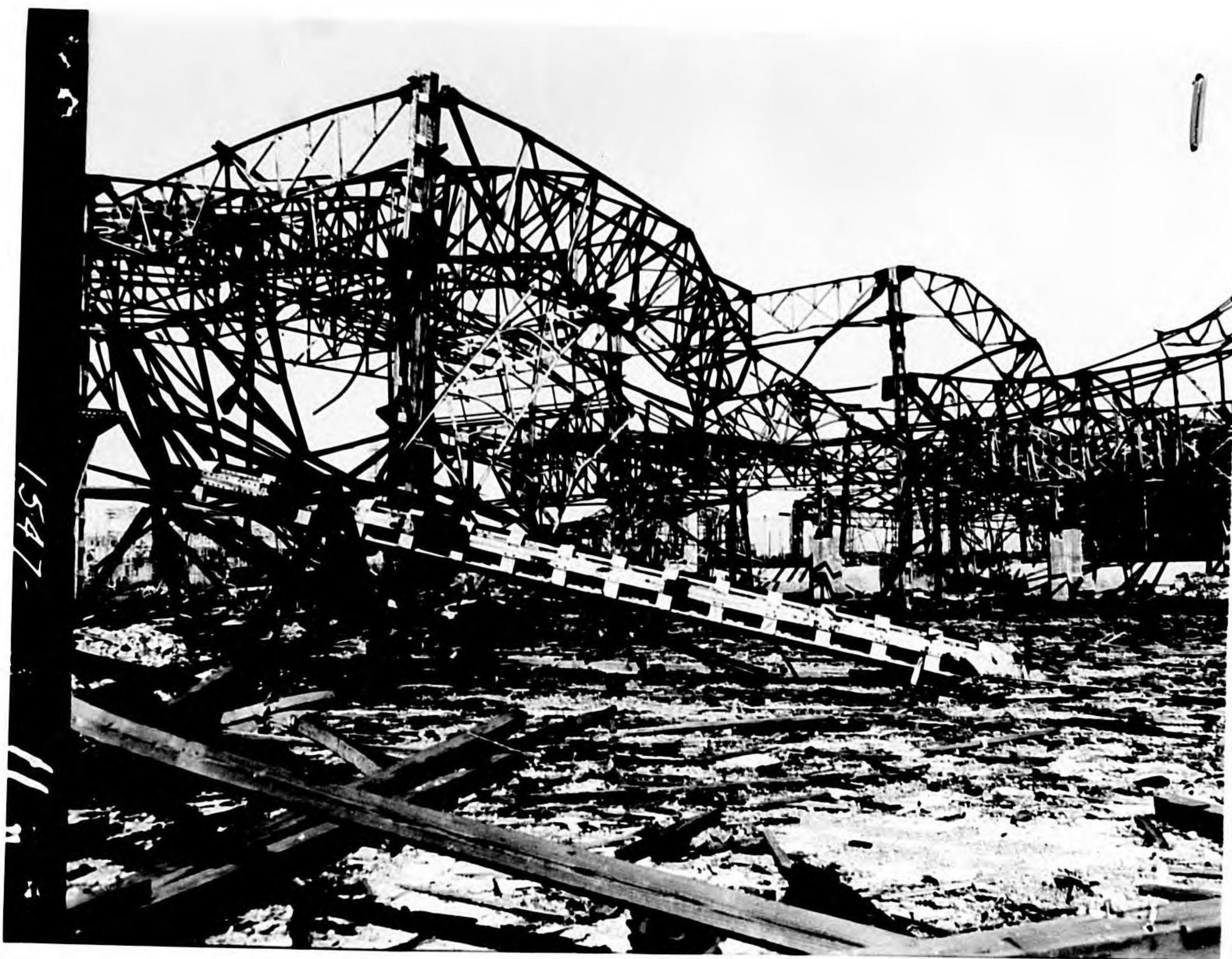
Photo 6 - Bldg 4, Bomb 29, Interior Column blown over.
