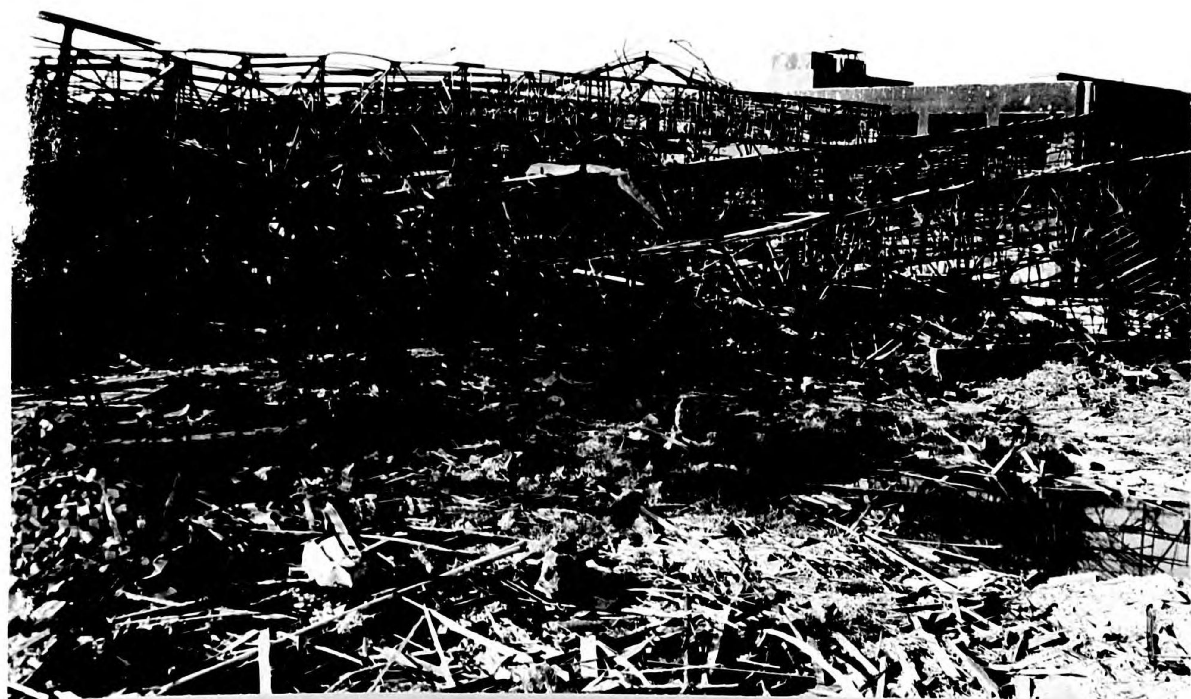
Photo 23 - Bldg. 27, Bomb 12, DAMAGE CAUSED BY NEAR MISS.
