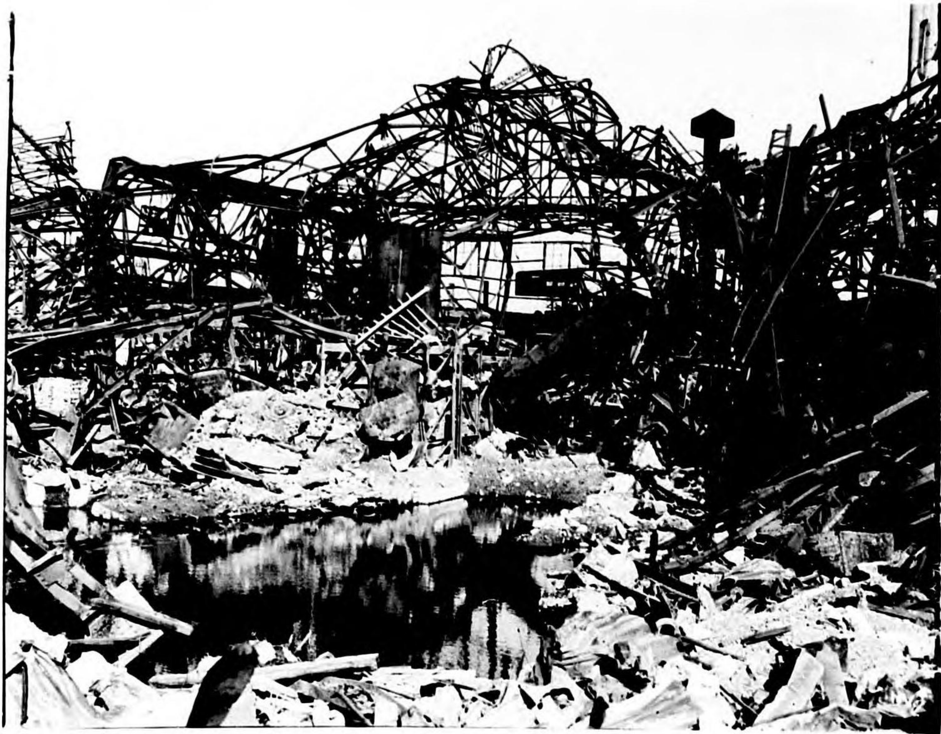
Photo 7 - Bldg. 14. Bomb 43. Damage to furnace and equipment.
