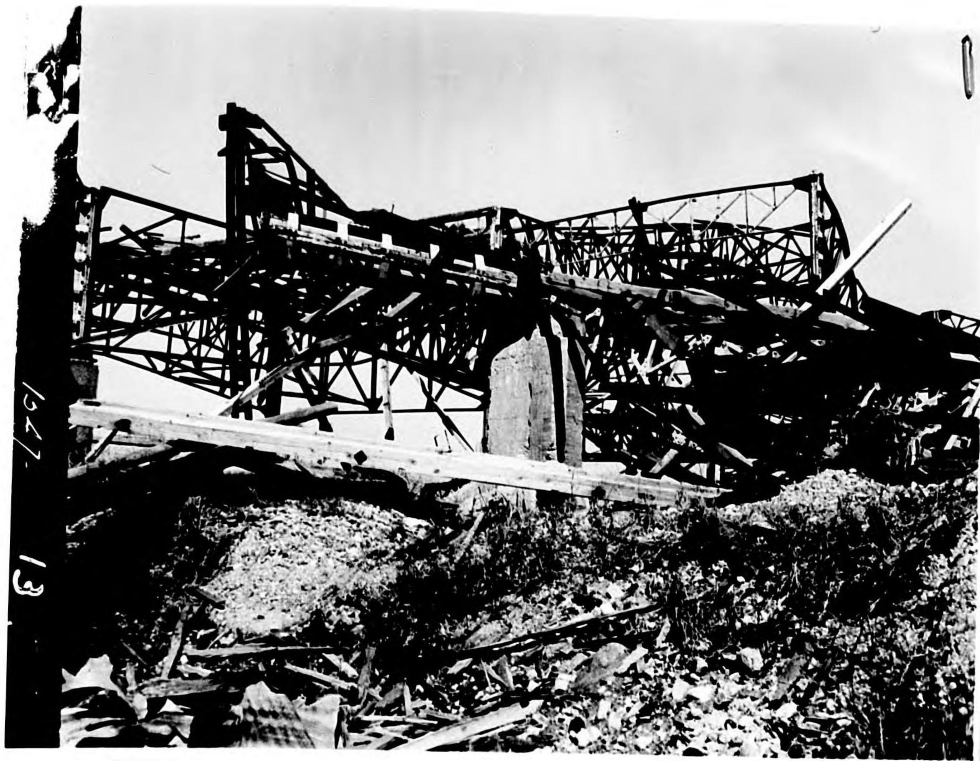
Photo 9 - Bldg. 4, Bomb 79, Exterior Columns blown over
