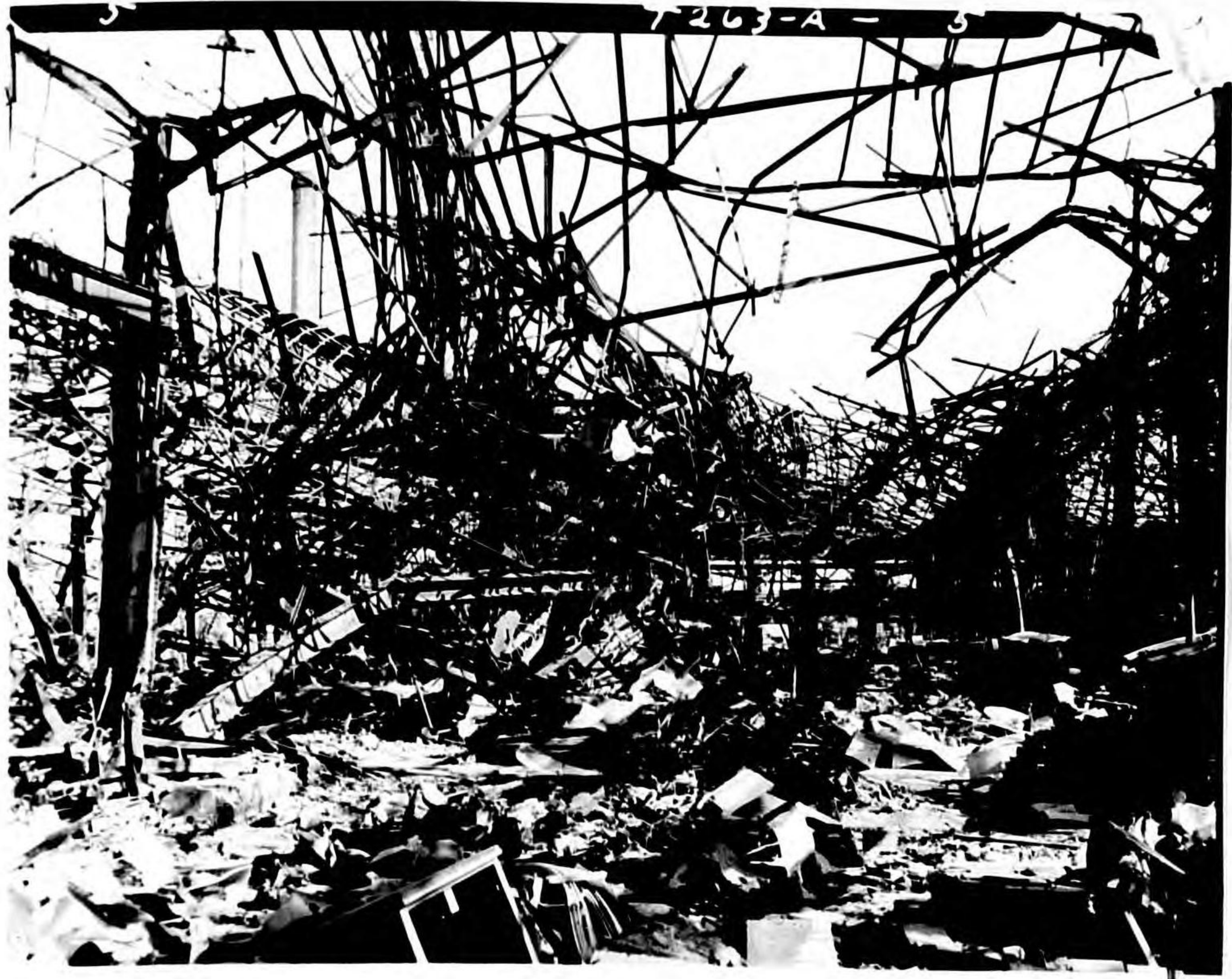
Photo 9 - Bldg. 64, Bomb 5. Severe damage.
