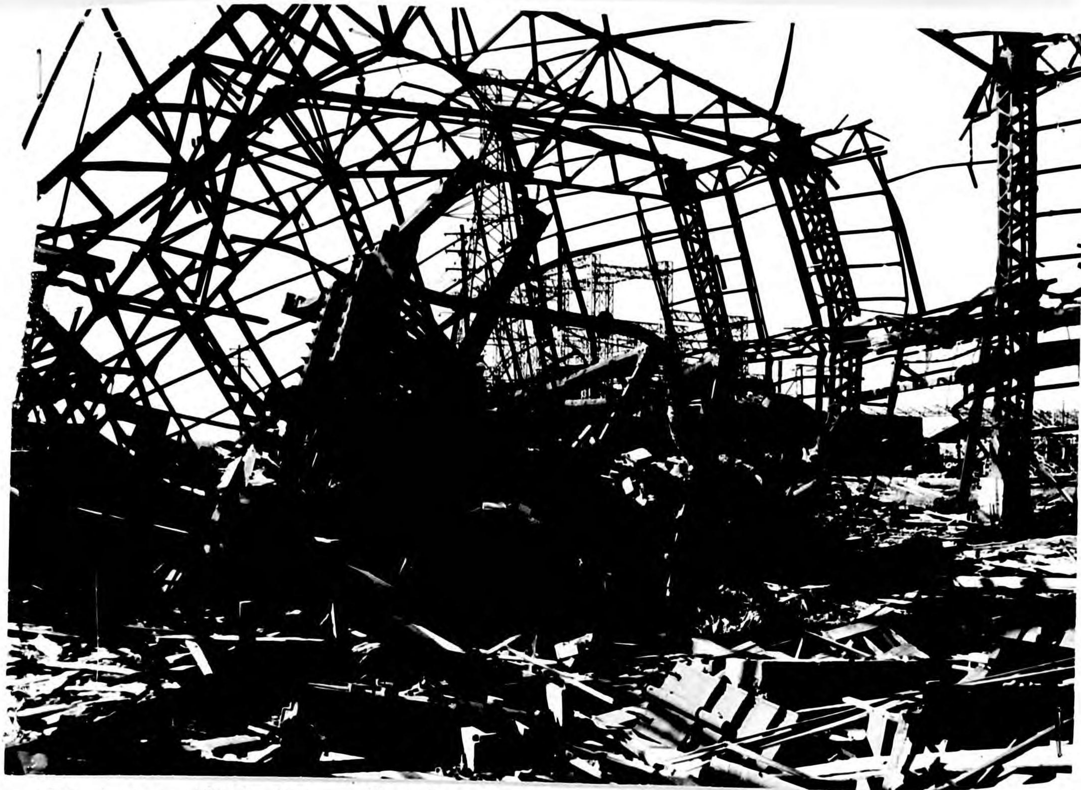
Photo 25, Bldg 132, Bomb 23, Boiler blown over.
