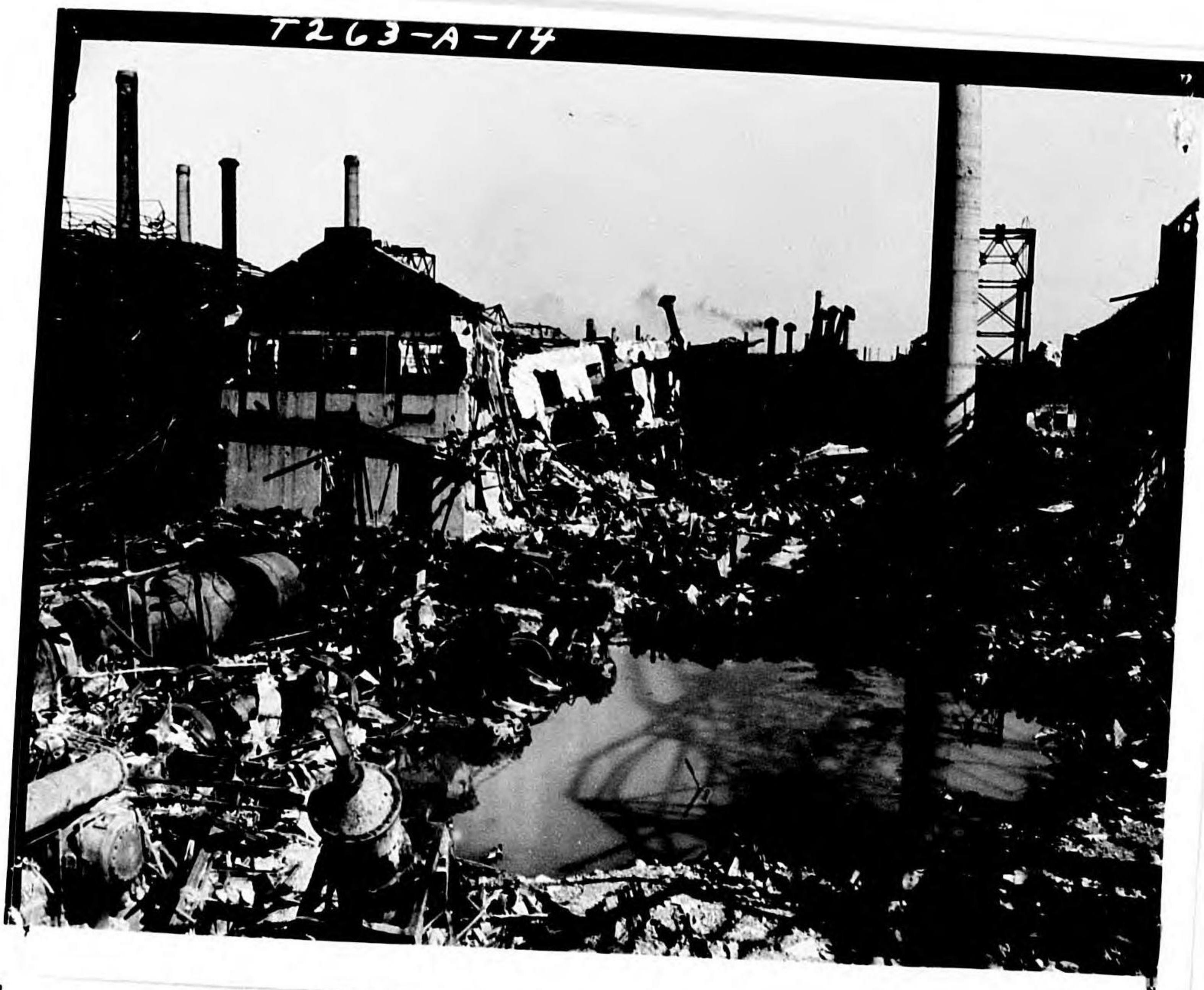
Photo 20 - Bldg. 62, Bombs 31, 32. Crushed buildings. 96
