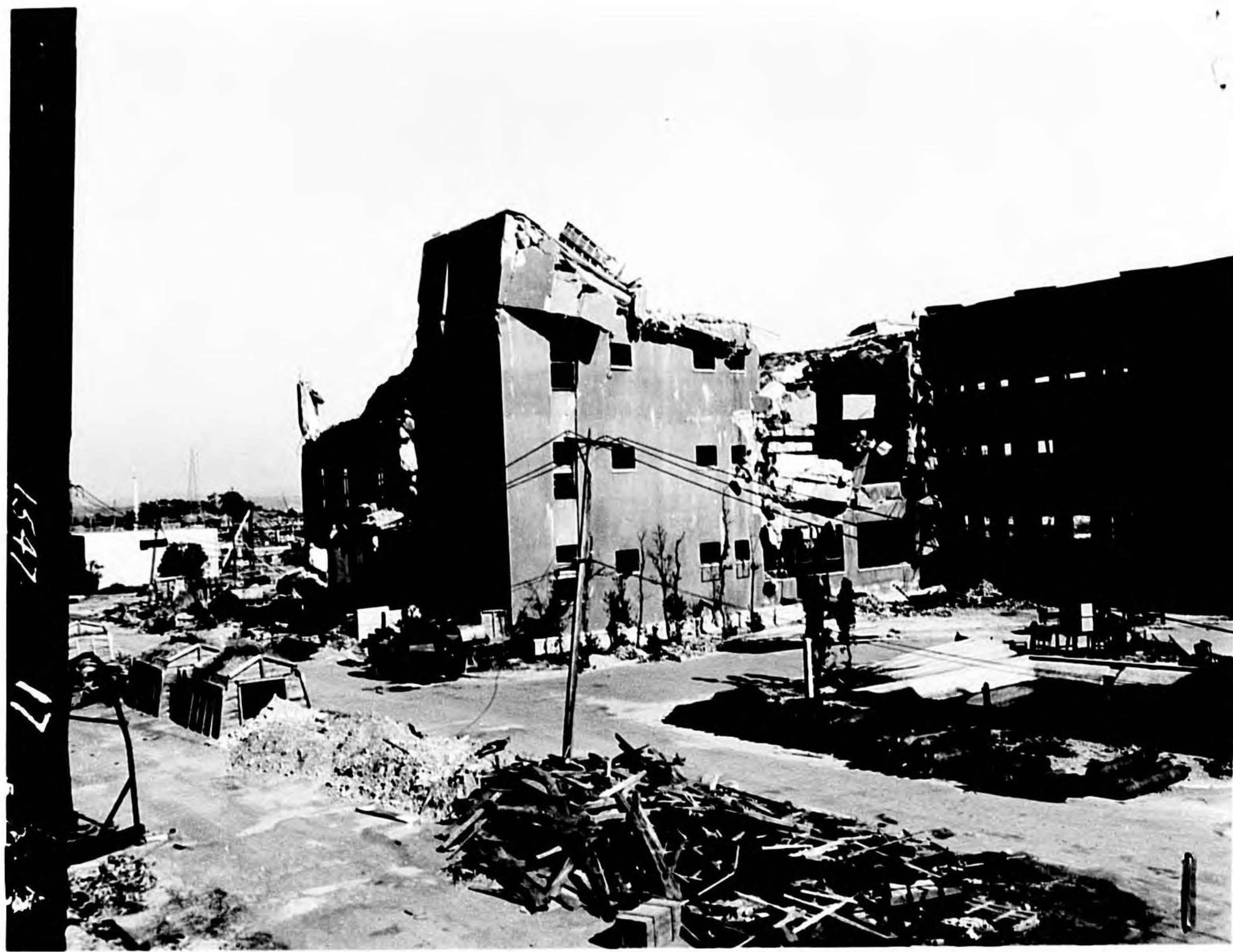
Photo 10, Bldg. 8, Bombs 45 and 46.
