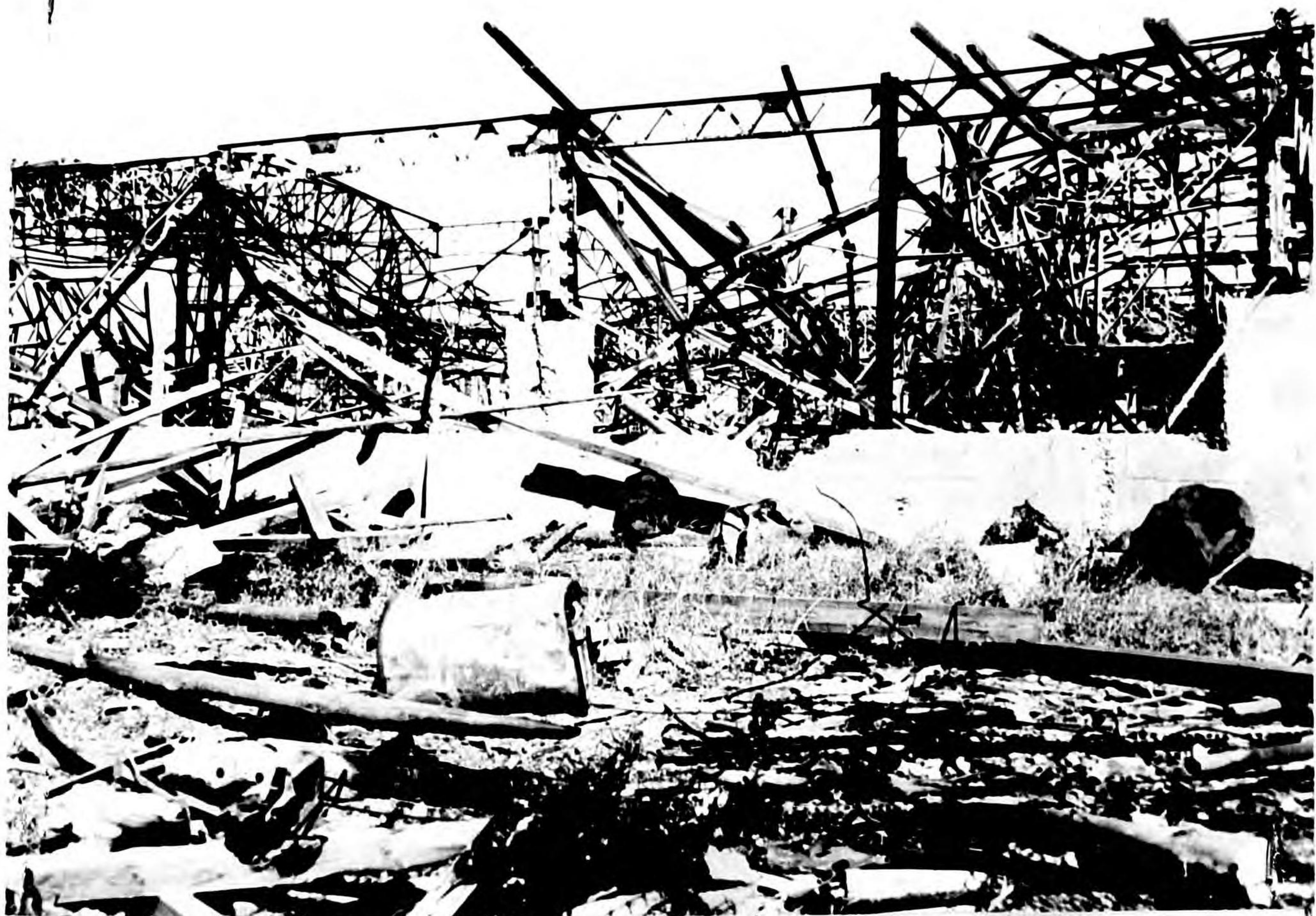
Photo 4 - Bldg. 4, Bomb 79 GENERAL VIEW. 38
