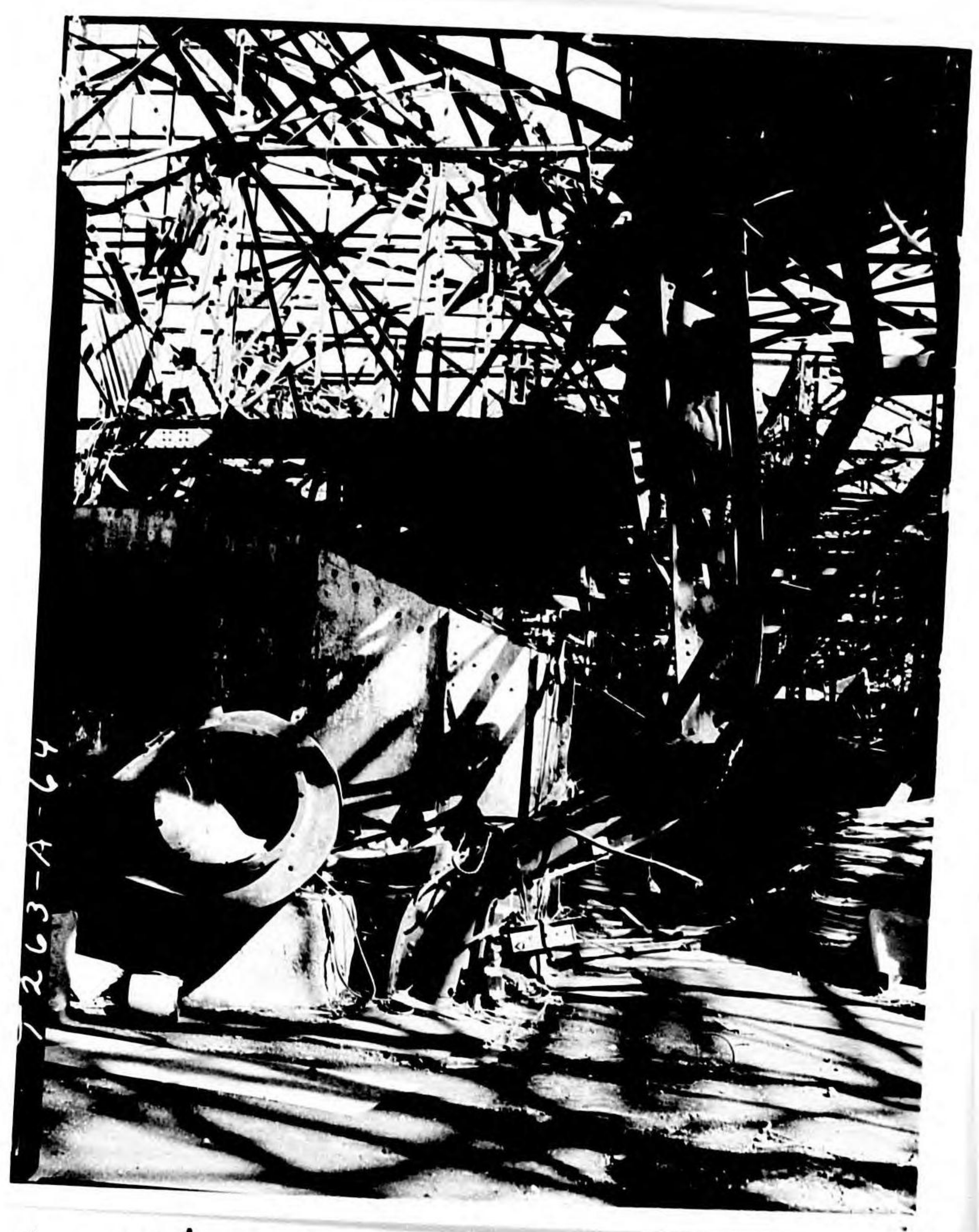
Photo 6 - Bldg. 14, Bomb 43. Column damage.
