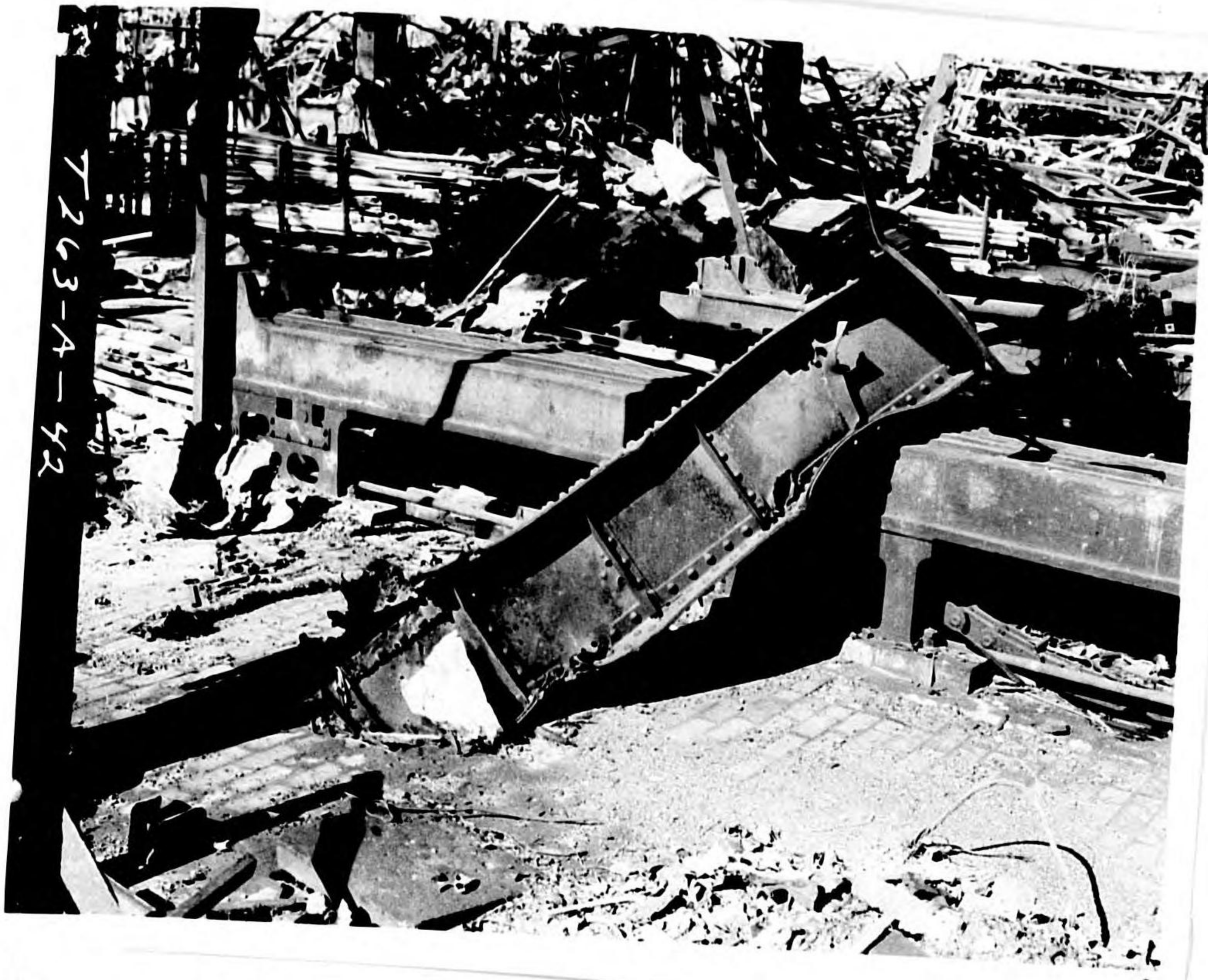
Photo 19 - Bldg. 51, Bomb 90. Detail of girder.
