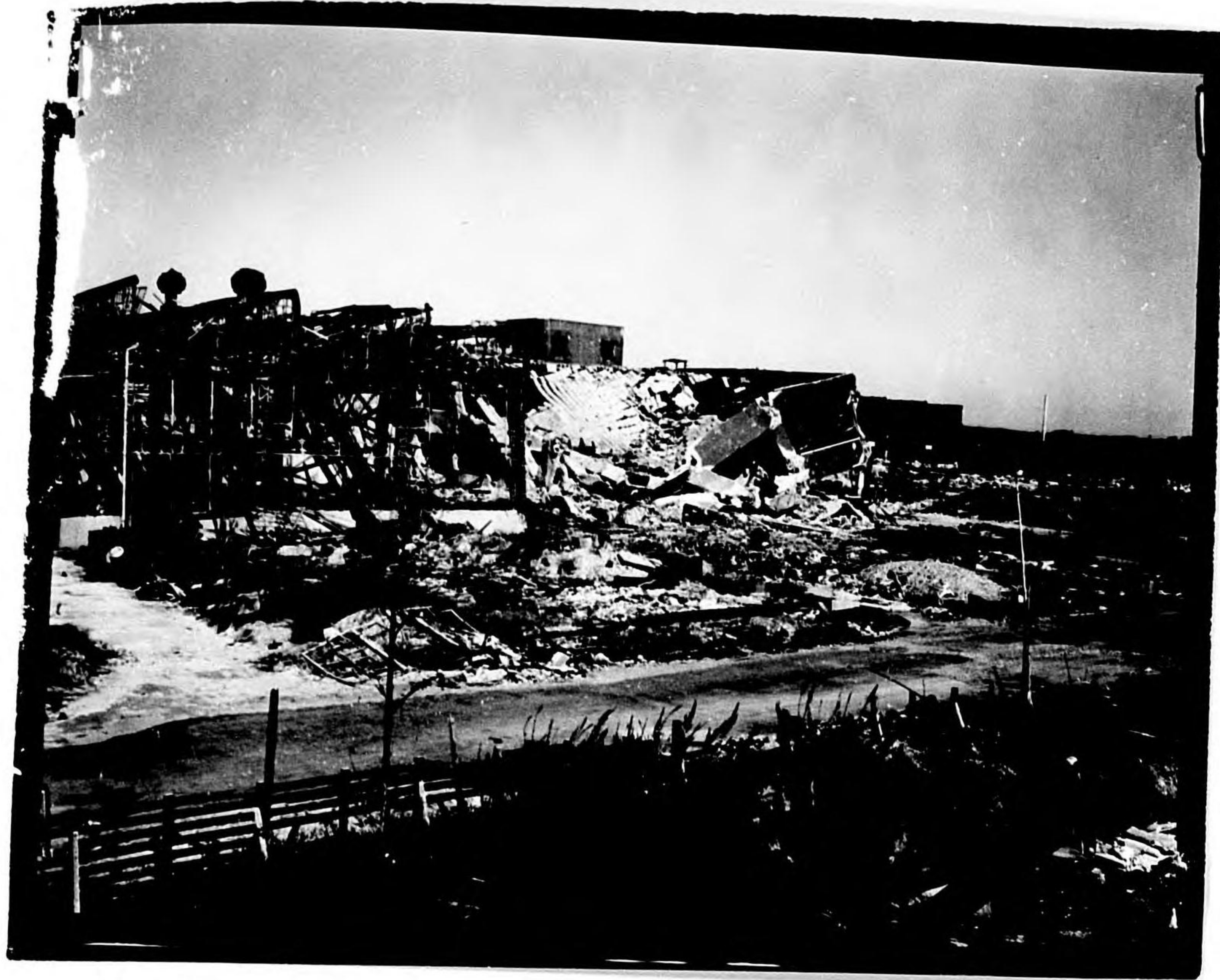
Photo 13, Showing damage to Bldg 23 and Bldg 12 by Bomb 15.
