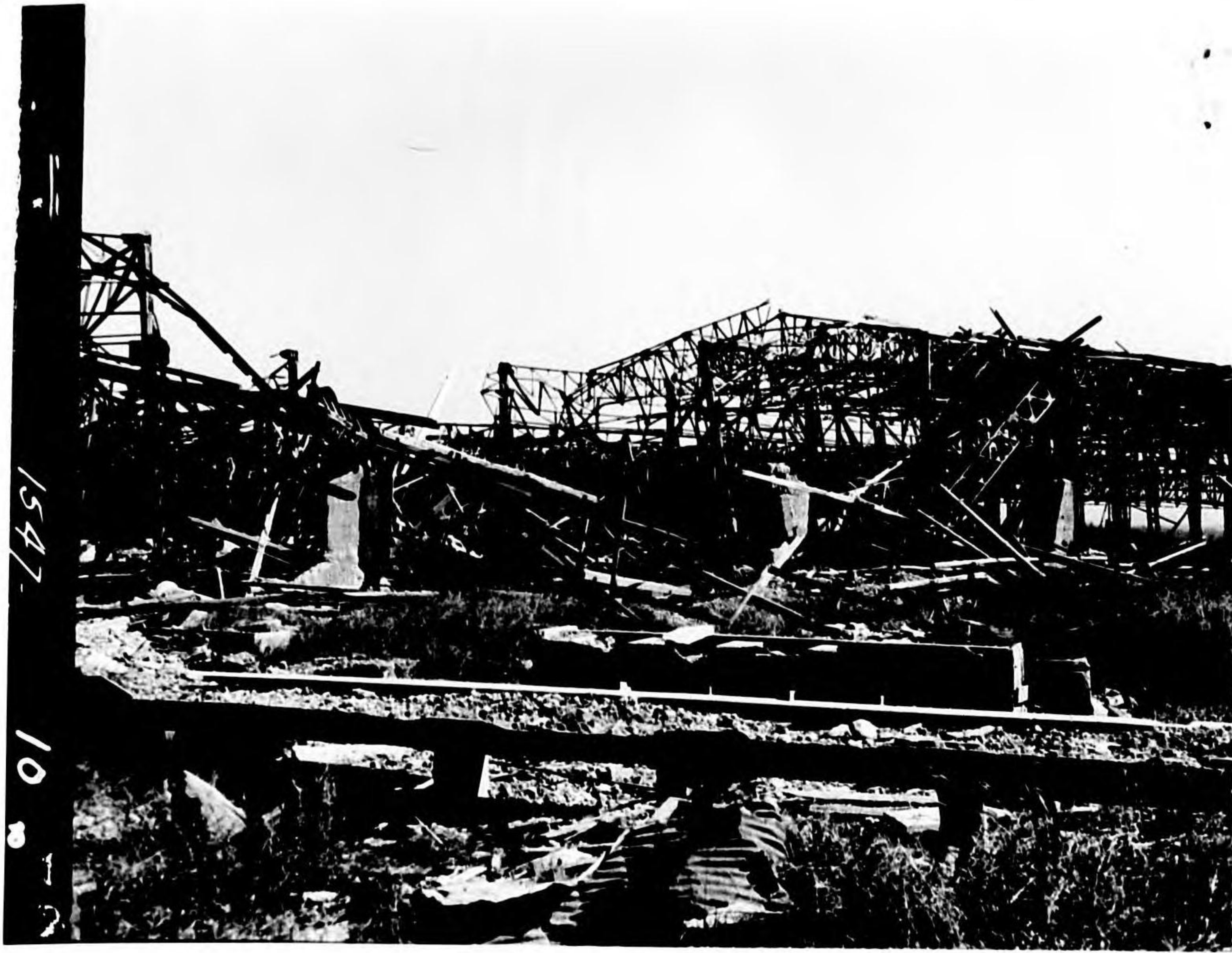
Photo 5 - Bldg 4, Bomb 29, General view.
