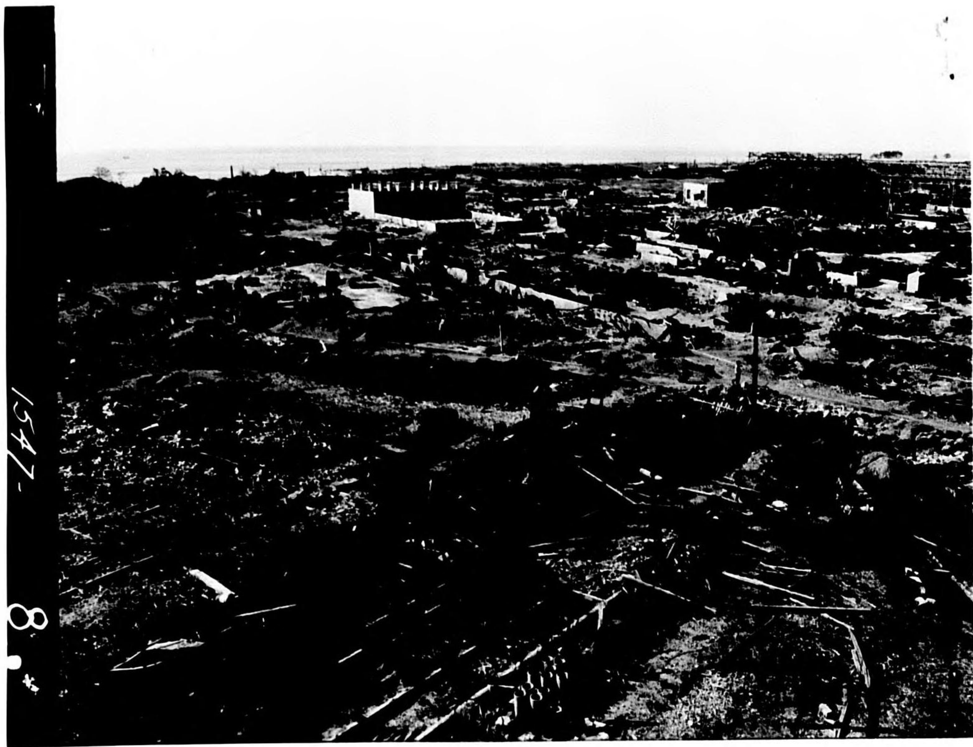
Photo 29- Overall view of fire damage caused by several 4,000-lb bombs.
