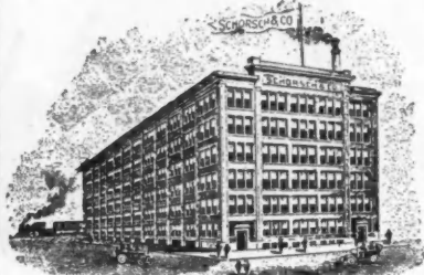
FACTORY 132 ND TO 133 RD ST. & BROOK AVE.
