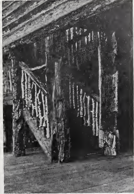
SIDE VIEW OF OUTSIDE RUSTIC STAIRWAY.
