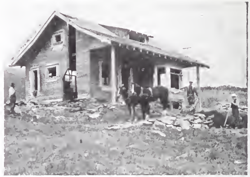
BUNGALOW IN PROCESS OF CONSTRUCTION.
