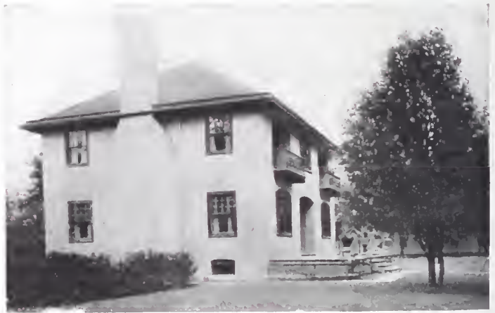
SIDE VIEW OF THE CONCRETE HOUSE AT SLEEPY EYE.
