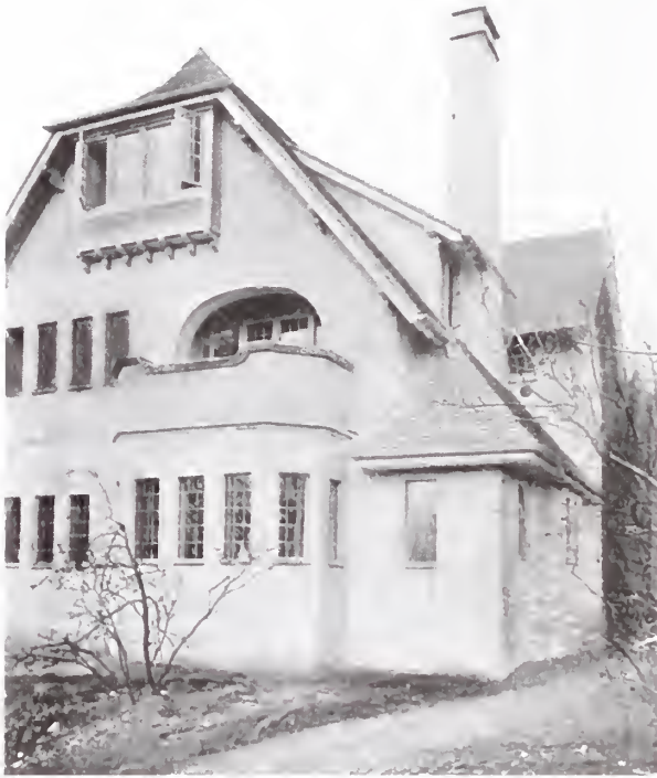
HOUSE AT CROYDEN IN SURREY, SHOWING BALCONY IN SECOND STORY.
