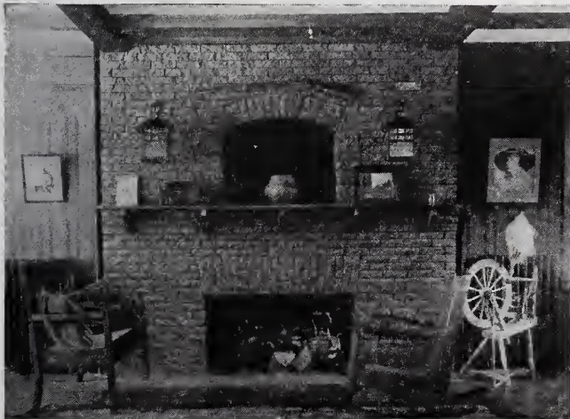
WELL-CONSTRUCTED FIREPLACE IN LIVING ROOM.
