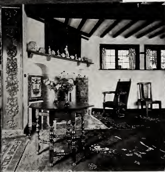
THE LIVING ROOM IN THE HOUSE AT NEWTON, THE WINDOWS PLACED SO THAT THE UTMOST LIGHT IS AFFORDED AND YET HIGH ENOUGH IN THE WALL TO AVOID GLIMPSES INTO NEIGHBORING HOUSES.
