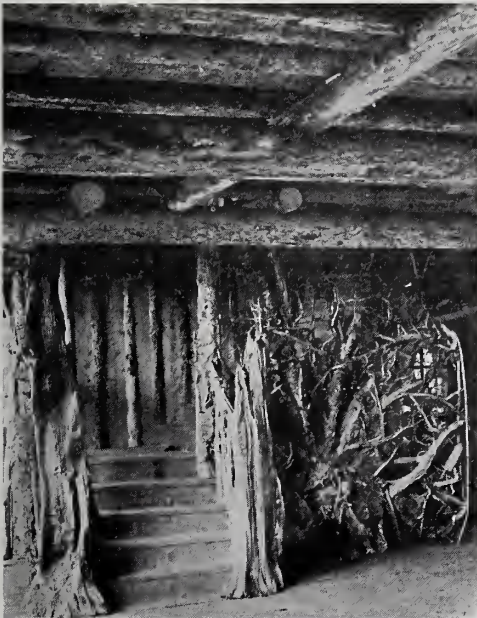
TREE STAIRWAY AND ROOT SCREEN IN THE FOREST HOUSE.
