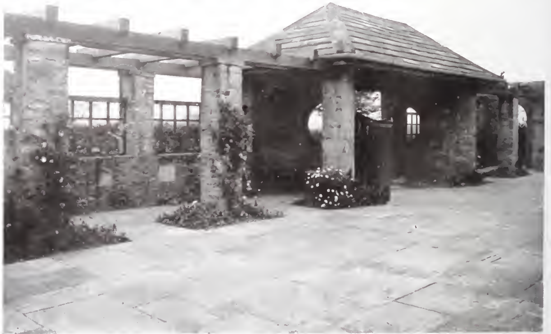
THE SOUTH AND GARDEN SIDE OF "WHIRRIESTONE," SHOWING GRACEFUL ROOF LINES. MAIN ENTRANCE: GATEWAY AND PERGOLA AT "WHIRRIESTONE."
