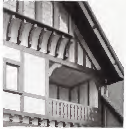
RECESSED BALCONY AT "SOMERSBY," BUXTON, DERBYSHIRE.
